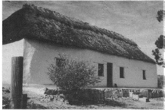
Fig 3: Groenfontein, Piquetberg. The front of a \perp -plan house, built as a replica of the original Groenfontein dwelling. Note the lintels and the ridge-capping of bundles of thatching-grass pulled up by the roots and placed roots uppermost. James Walton 1965
