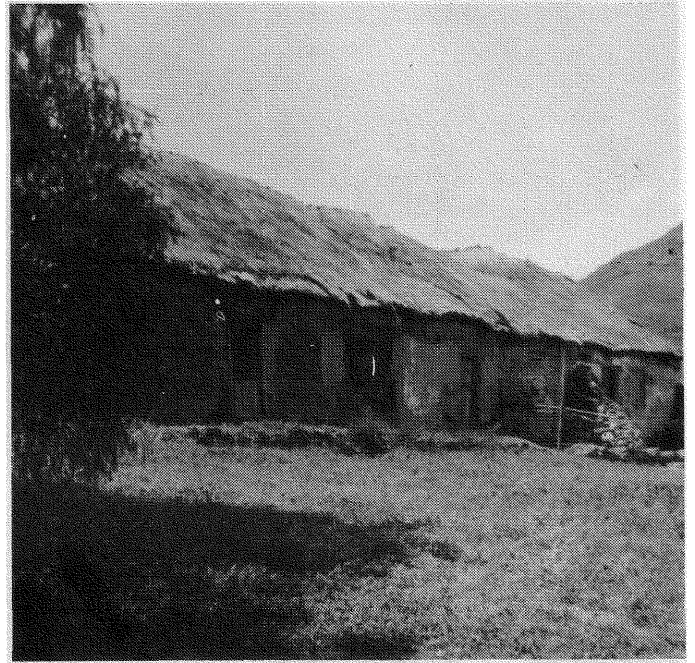
Fig 13: Eselshoek. The house painted by Poortermans as it appeared in 1965. Windows blocked up and an extension added on the right. Walls built up of layers of clay mixed with chopped straw.
