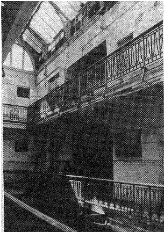
Gallery of Somerset House, view taken looking northward (towards Fox street). Note the glass bricks incorporated in the upper gallery floor.
