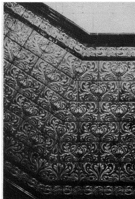
Tiling on the walls in the basement.
