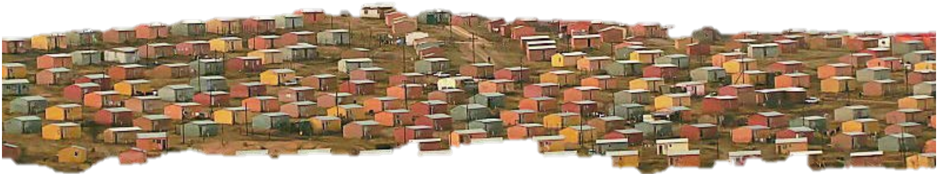
Figure10: Typical subsidised housing in South Africa illustrates the resultant poor quality living environment and lack of variation in typology ( www.trekearth.com )
