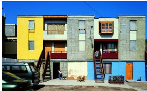
Figure 43: View of Quinta Monroy with the extensions done by the residents (www.archdaily.com)
