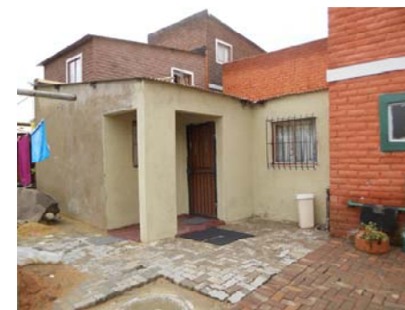
Figures 103: Extensions to the buildings by the homeowners (Osman & Davey 2011:4)
