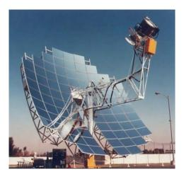
Figure 1.2 Parabolic dish concentrator for a Stirling engine (Image extracted from Pitz-Paal, 2007).
