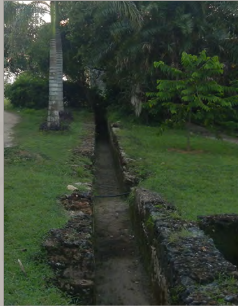
Fig. 71: Original aqueduct fabric still visible on site (Author, 2013).
