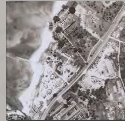
Aerial photograph of Mtoni Palace with Mtoni Marine being constructed [1989]
