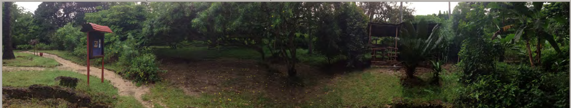
Fig. 77: Photograph showing the break in the historic aqueduct (Author, 2013).
