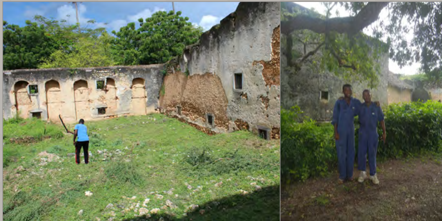
Fig. 89: The maintenance team (Author, 2013).
