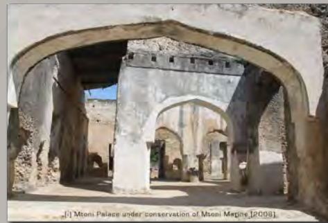
Mtoni Palace under conservation of Mtoni Marine [2008]
