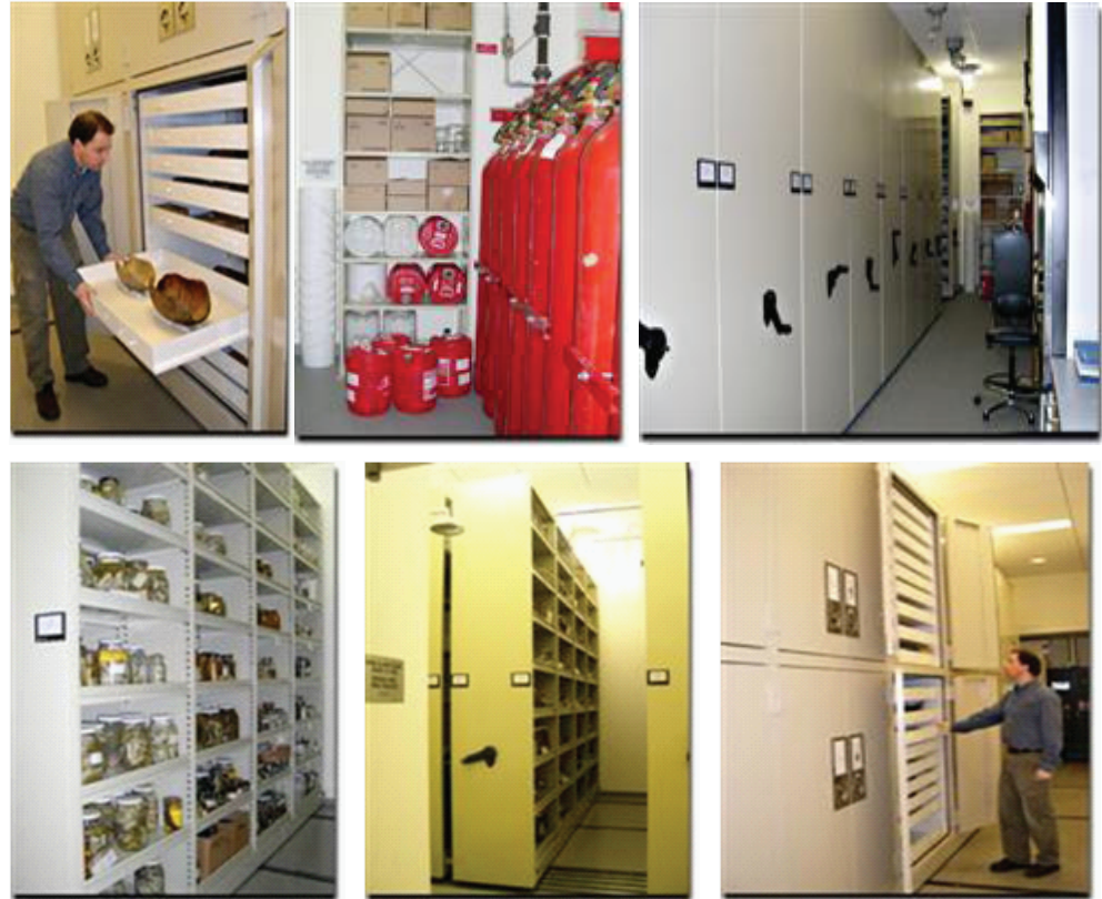
Figure 71: Inergen fire suppressing gas system and spirit storage, http://bgbaseserver.eeb.uconn.edu/floorplan/index.htm
