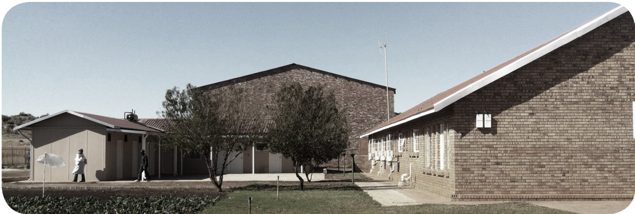
1.7: Photograph of the site arrangement at Steve Tshwete PHC. (Author, 2014).
