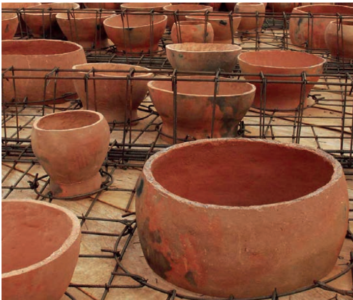
Figure 2.18. Installing pots in school library, Gando Burkina Faso (Kere Architecture [Sa])
