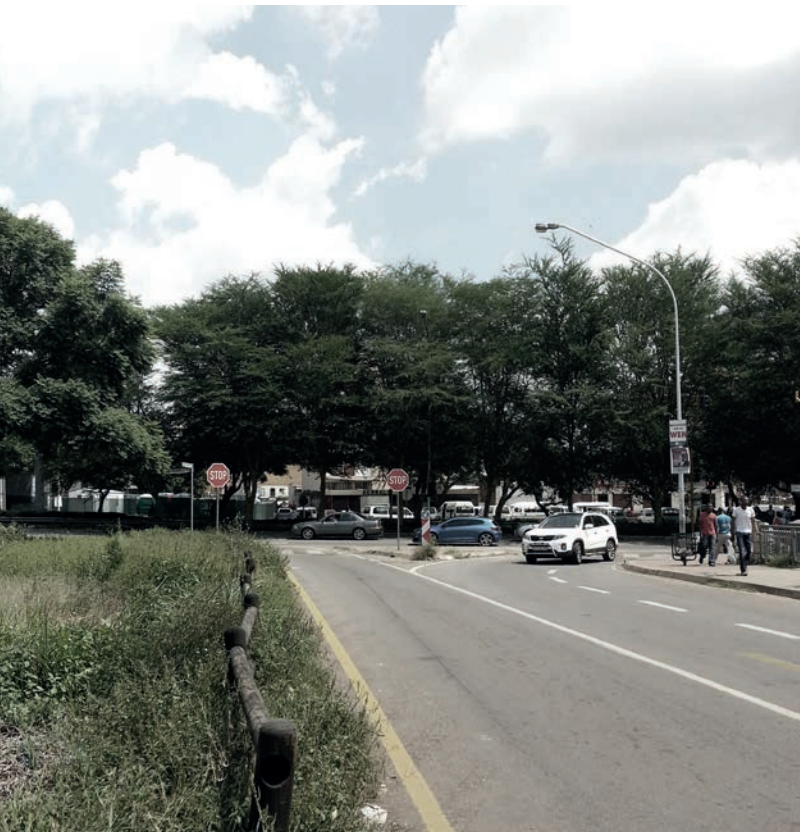
Figure 3.41. Panoramic view of site, towards Nelson Mandela Drive
