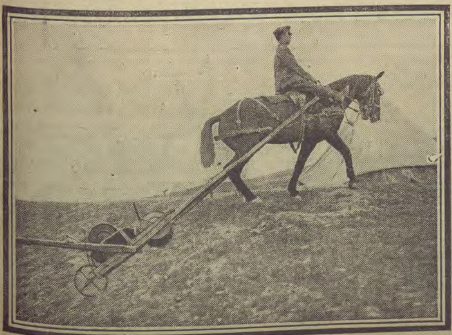
How the British Signal Corps lay field telephones along the rugged hill frontiers at Salonika.
