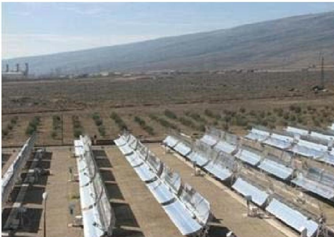
Figure 4 A view of collectors' field
