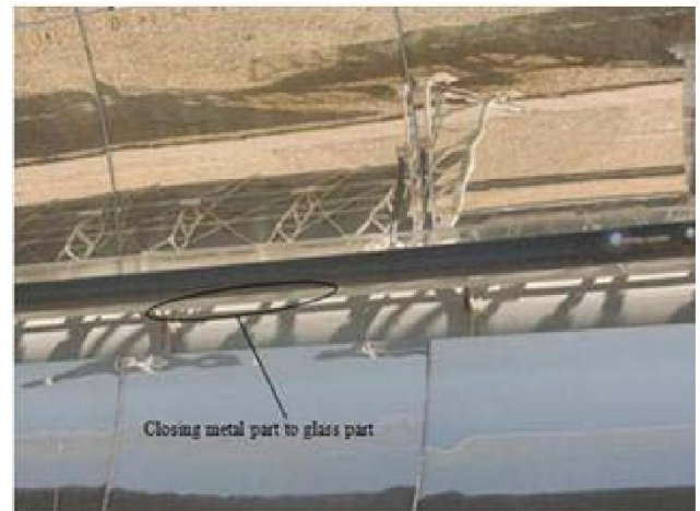
Figure 9 Closing of metal part of receiver tube to glass
