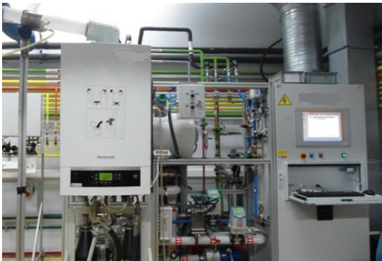
Figure 12 Special test rig for comfort and efficiency tests of combi boilers
