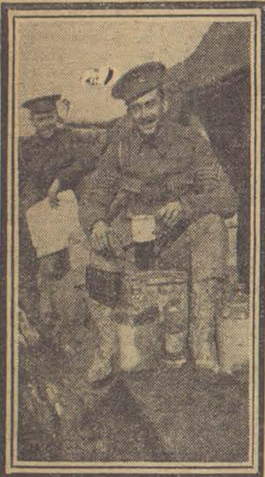
London Rifle Brigade men in the trenches which they held unbroken from December to March.
