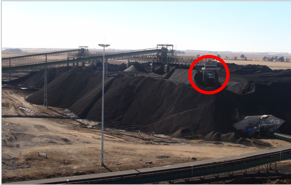
Figure 2.2: Dozer activity on an over-filled stock pile.
