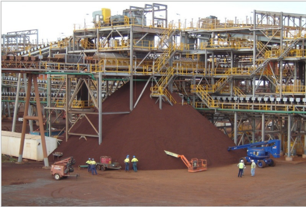
Figure 1.2: Unforeseen loads exerted on support structures.
