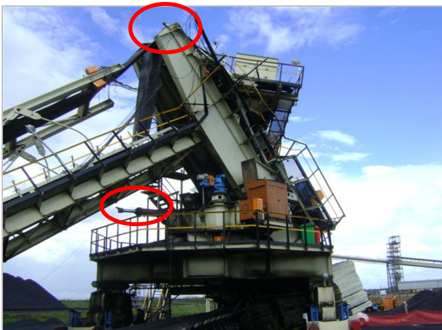
Figure 5.7: Collapsed machine with luffing cylinder and main boom connection highlighted.
