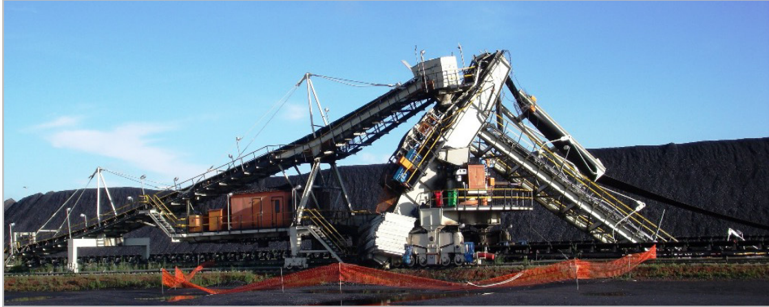
Figure 5.3: Collapsed stacker viewed from the south.
