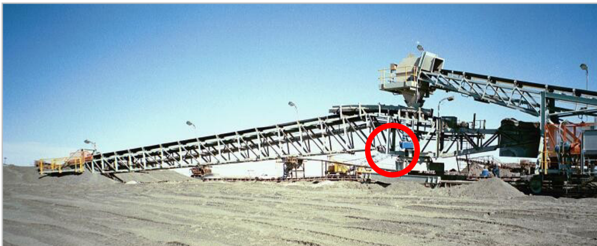
Figure 3.2: Waste spreader failure.
