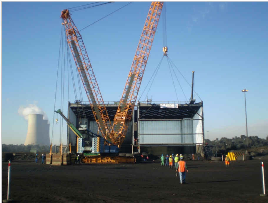
Figure 2.4: Major construction rigging, 80 ton single lift.
