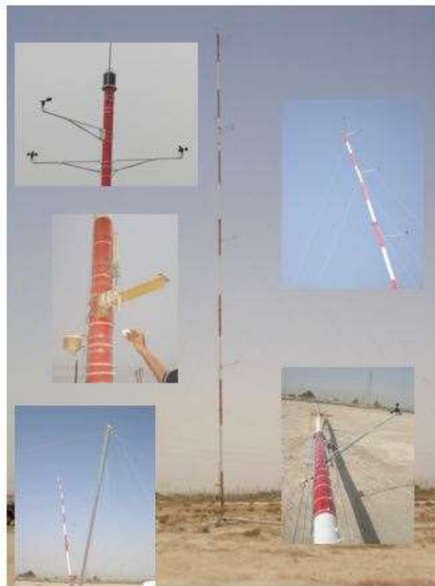
Fig. 2. Wind and meteorological data measurement tower.
