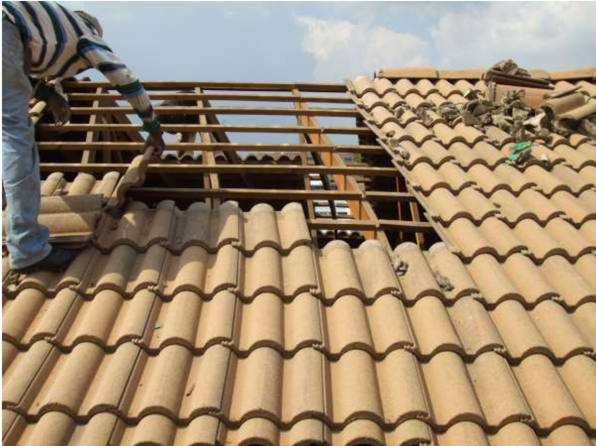
Photograph 1: This shows the buckling of the top chords of a timber trussed roof where no bracing has been supplied.
