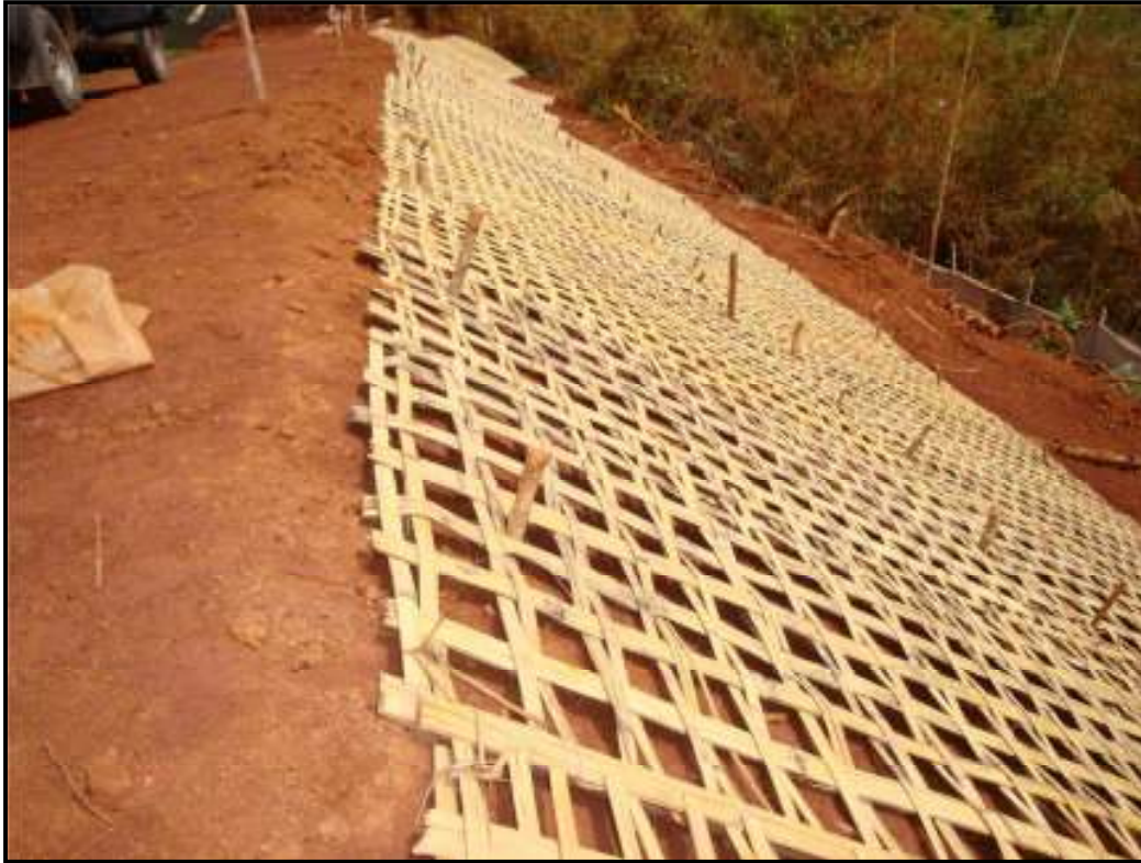
Figure 9.3 Woven geotextile mats in Madagascar
