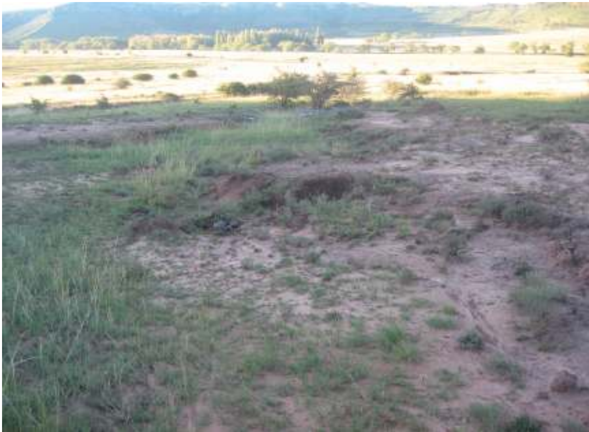
Figure 6.5 Erosion at Ladybrand site
