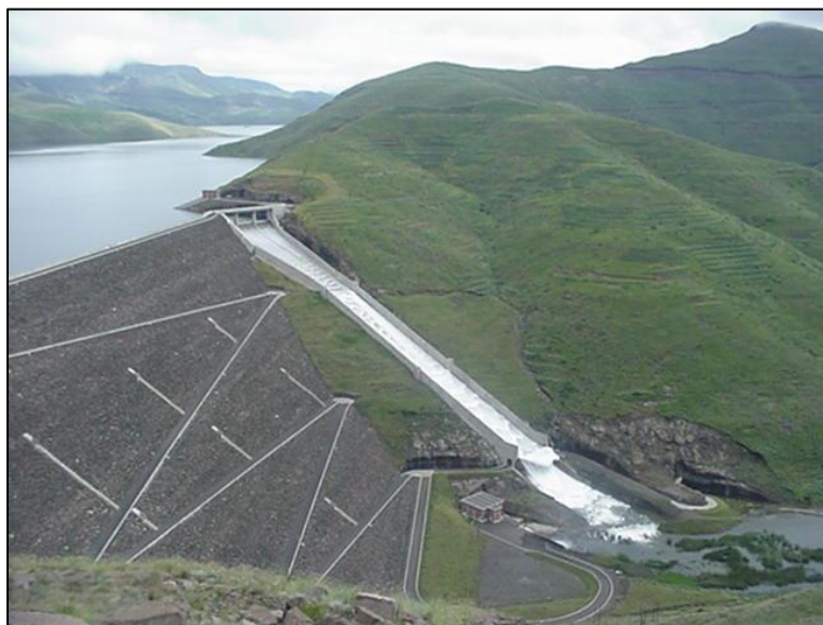
Figure 2-2: Mohale dam spilling February 2006 (International Water Power and Dam Construction, 2009)
