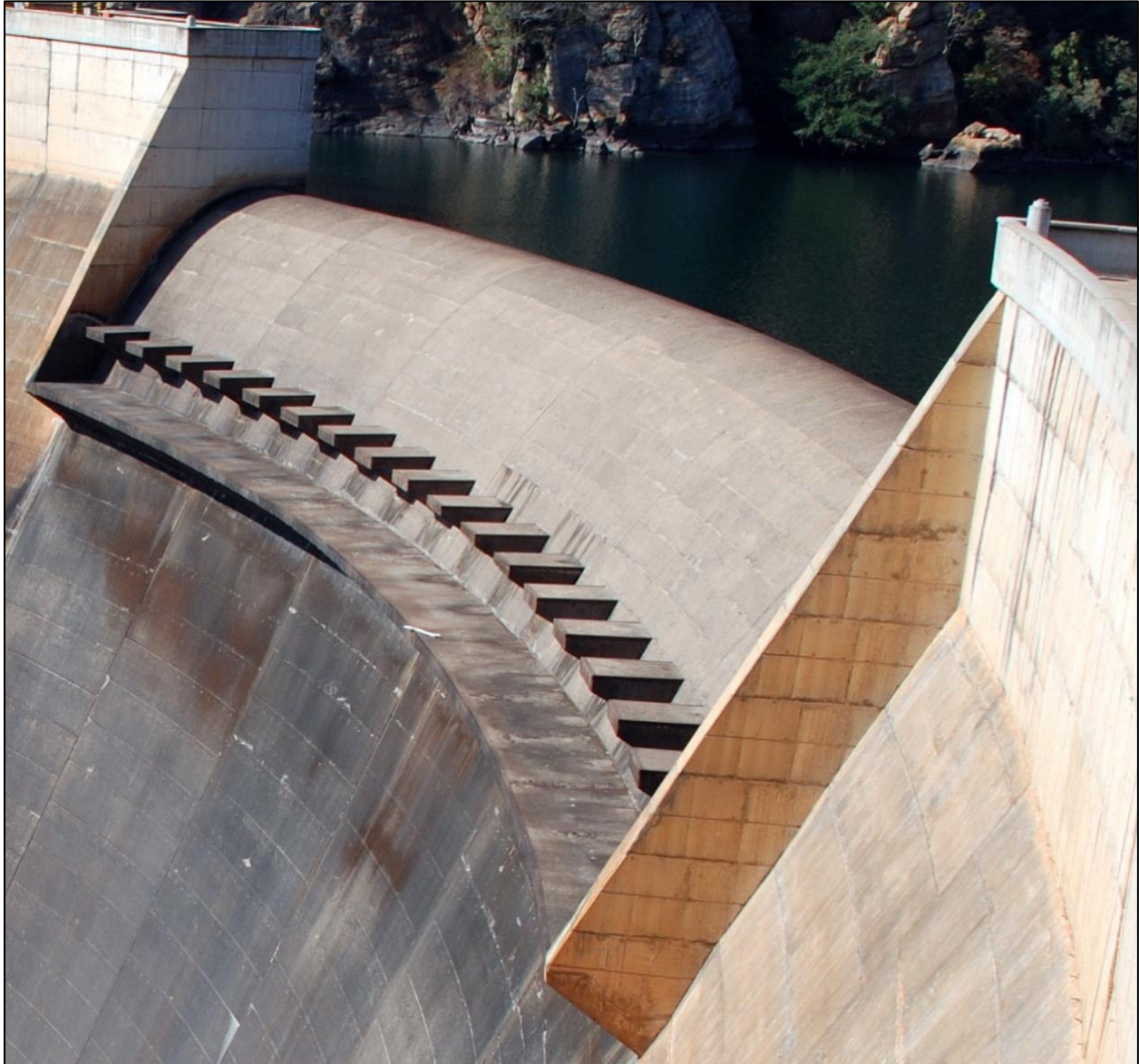
Figure 1-1: Blyderiverpoort Dam, Mpumalanga, South Africa (Ogee spillway with Robertson Splitters) (Yahoo! Inc., 2011)
