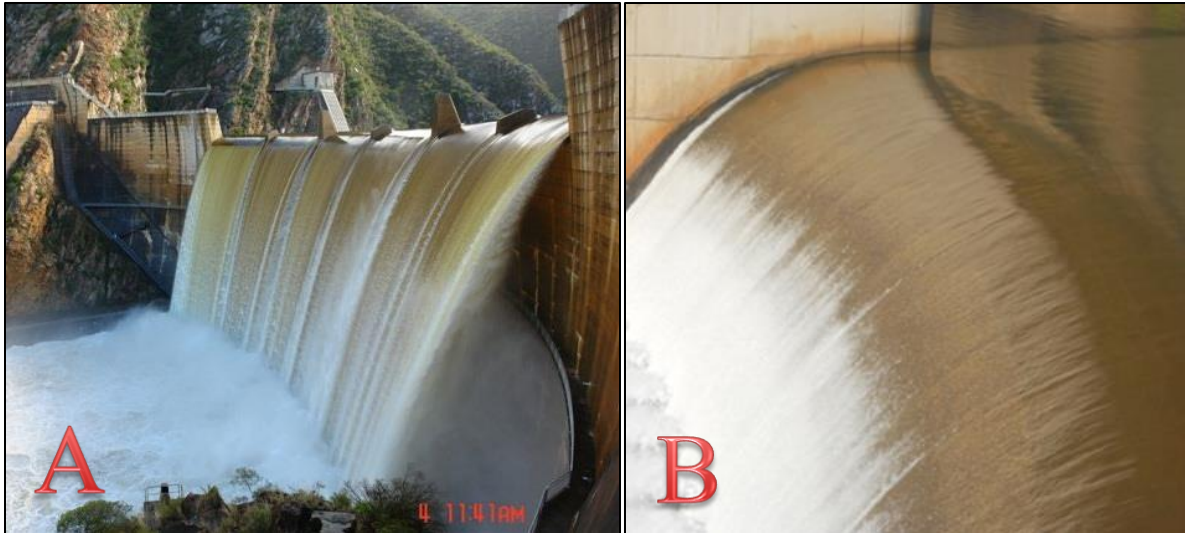
Figure 1-5: Free overfall spillway (Kouga Dam, Eastern Cape, A) and Ogee Spillway (Blyderiverpoort Dam, Mpumalanga, B)
