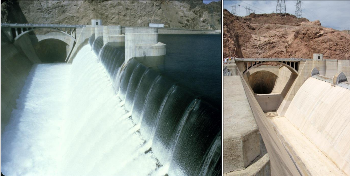
Figure 2-3: Hoover Dam side channel spillway overflowing 1983 (Wiltshire, et al., 2010)
