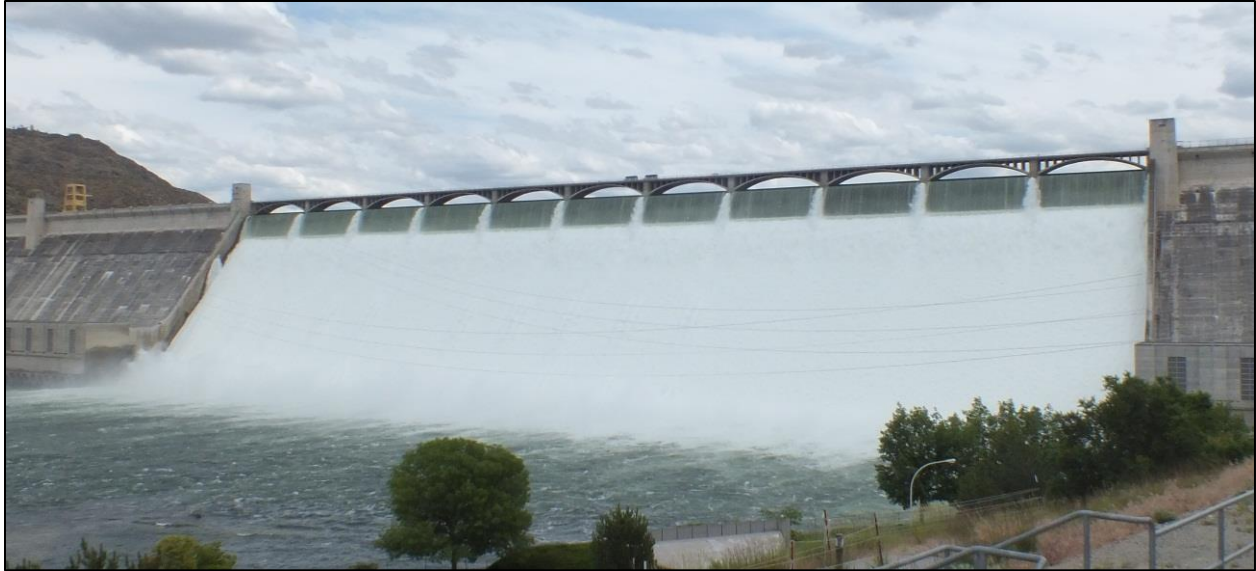
Figure 2-1: Grand Coulee Dam Ogee spillway spilling 2011 (Yahoo! Inc., 2011)
