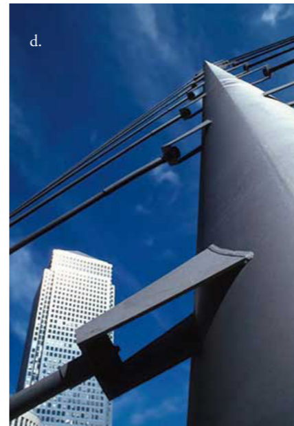
Fig.11.29 South Quay foot bridge, London by Chris Wilkinson with Jan Bobrowski & Partners (1997). Detail of top pylon/cable connection.
