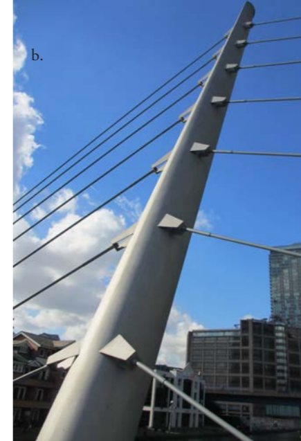
Fig.11.29 South Quay foot bridge, London by Chris Wilkinson with Jan Bobrowski & Partners (1997). Detail of top pylon/cable connection.
