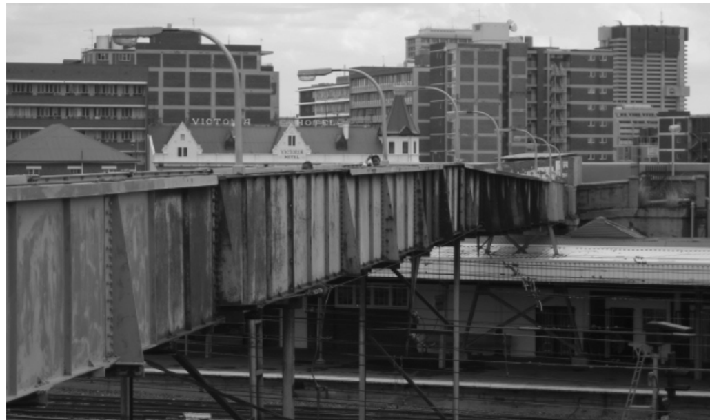
Fig.2.47 The existing pedestrian bridge providing the only physical link between Salvokop and the city, viewed from the original pedestrian bridge.
