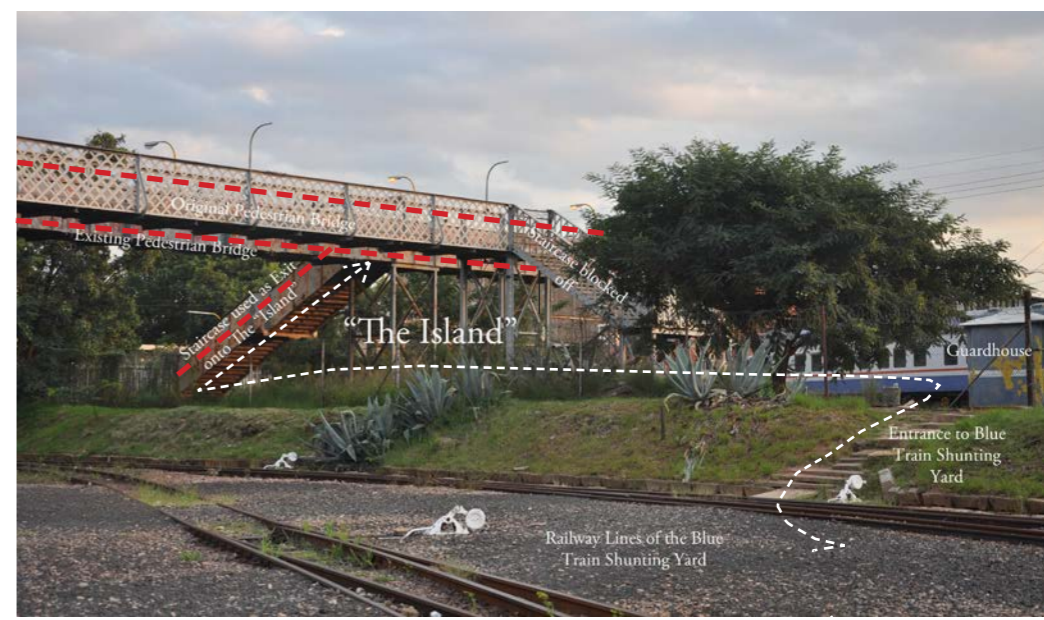
Fig.2.17 The "Island", viewed from the railway lines of the Blue Train Shunting Yard to the south east, indicating the position of the existing staircase and guardhouse.
