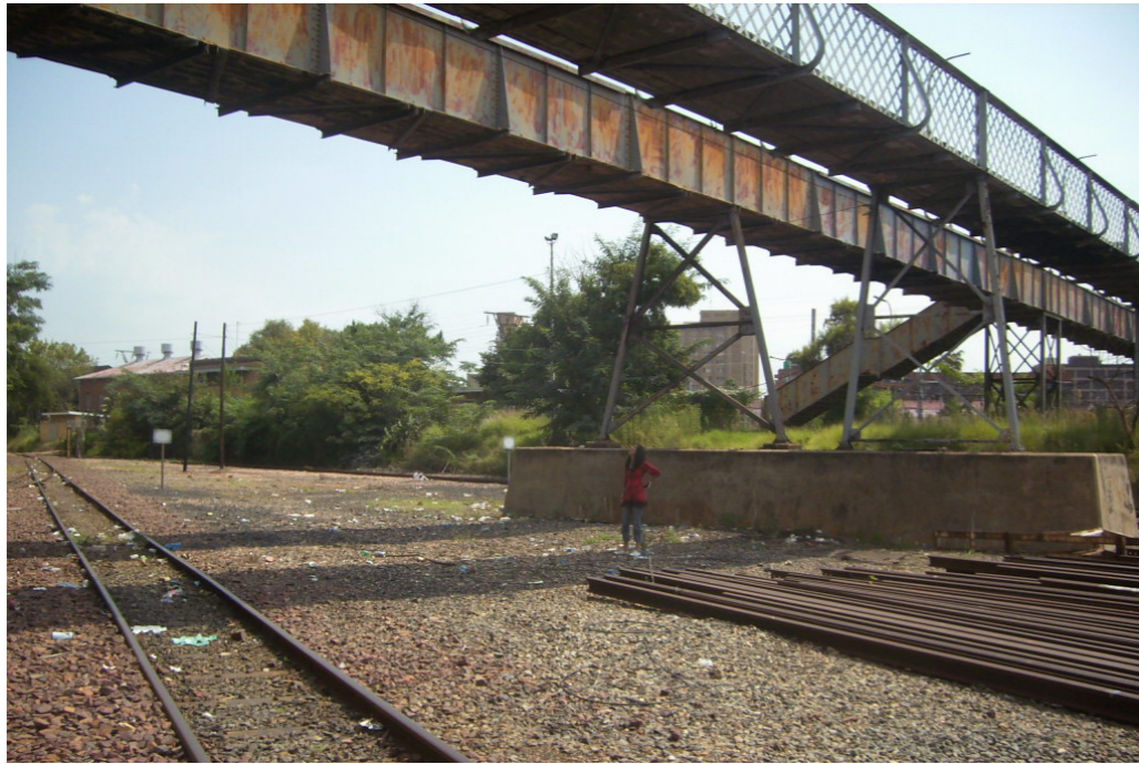
Fig.3.12 The existing and original pedestrian bridges viewed from below from the Blue Train Shunting Yard.
