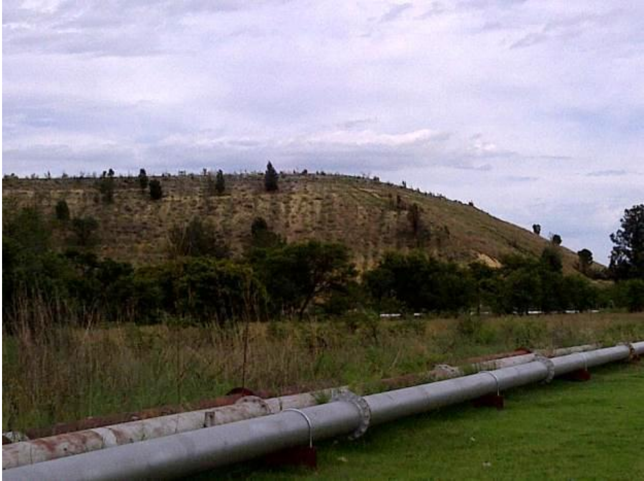
Figure 3.11: No. 3 Tailings dam
