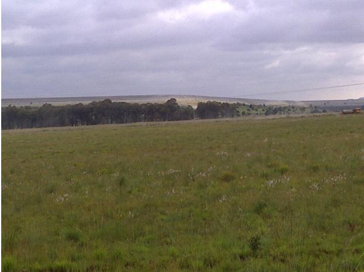
Figure 3.10: No. 1 and 2 Tailings dams
