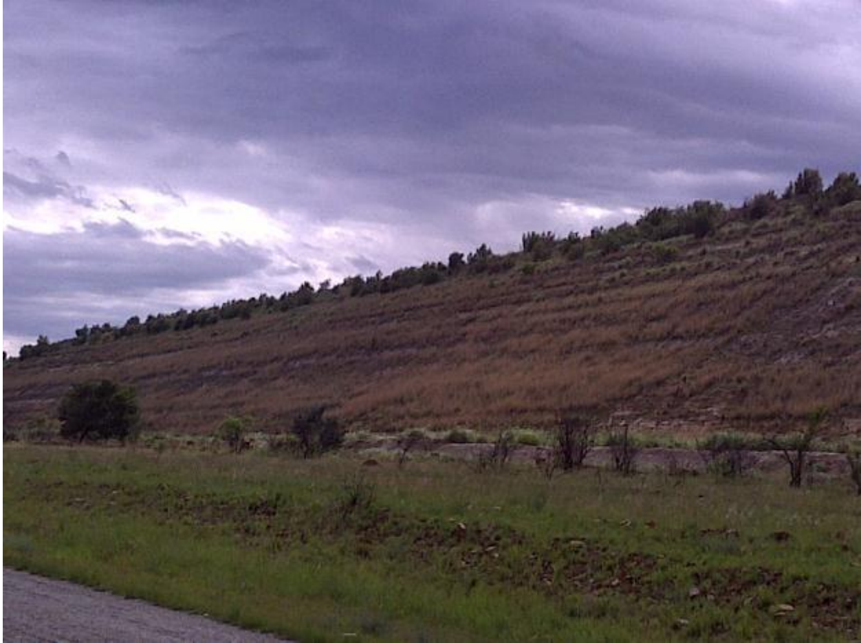
Figure 3.13: No. 5 Tailings dam
