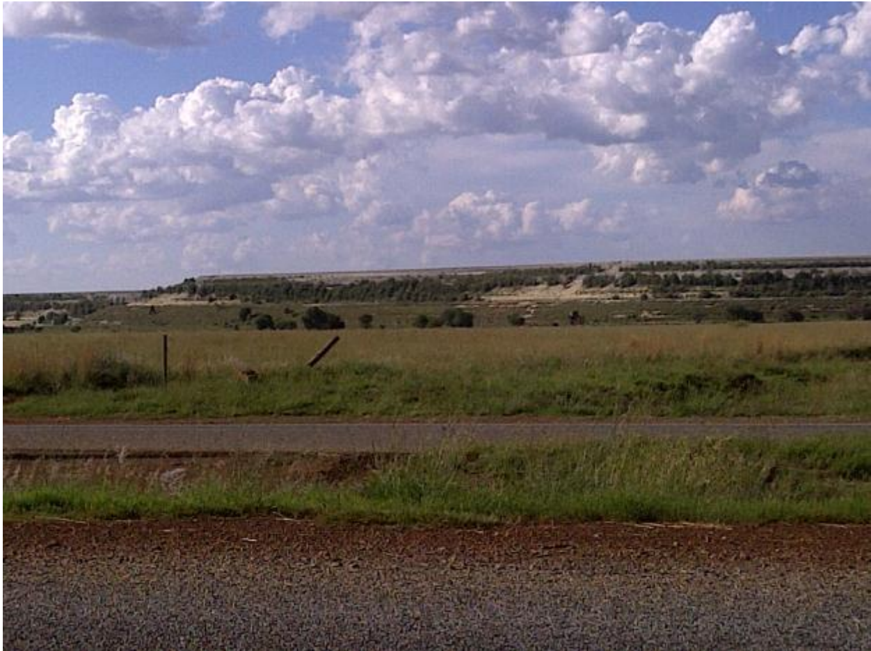
Figure 3.12: No. 4 Tailings dam
