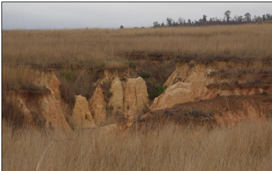
Figure 3-3: Sample suspected to be highly dispersive (13O3) with erosion gullies and piping structures.
