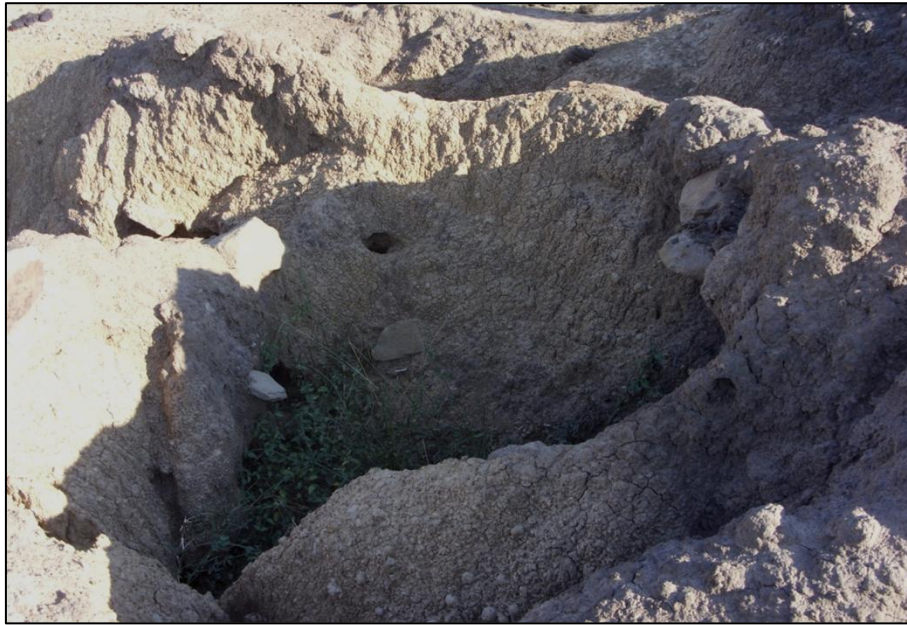
Figure 3-4: Sample expected to be highly dispersive (N2S2) with piping and tunnel features.
