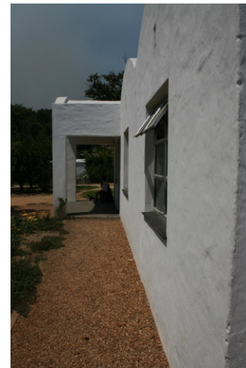
9. View looking east
