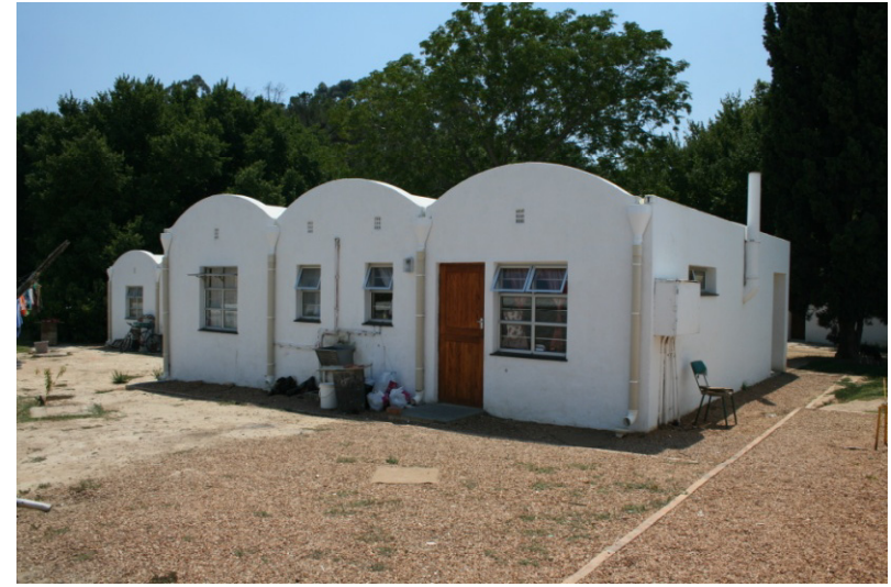
3. View of the south-east corner
