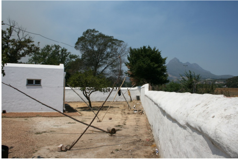
4. View of the yard looking east
