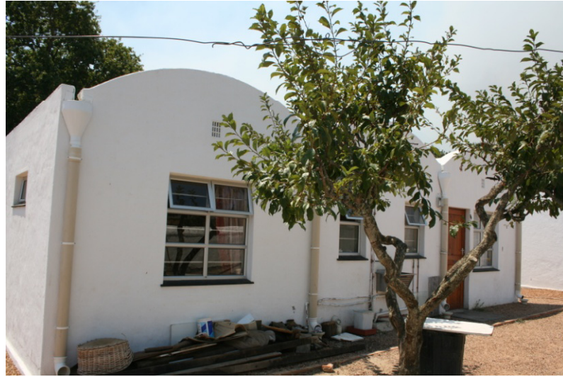
5. View of the southern facade
