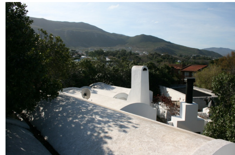
10. View over the roof looking north-east
