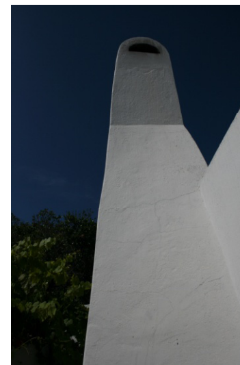
9. View of the chimney
