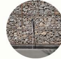
dolomite gabion walls
