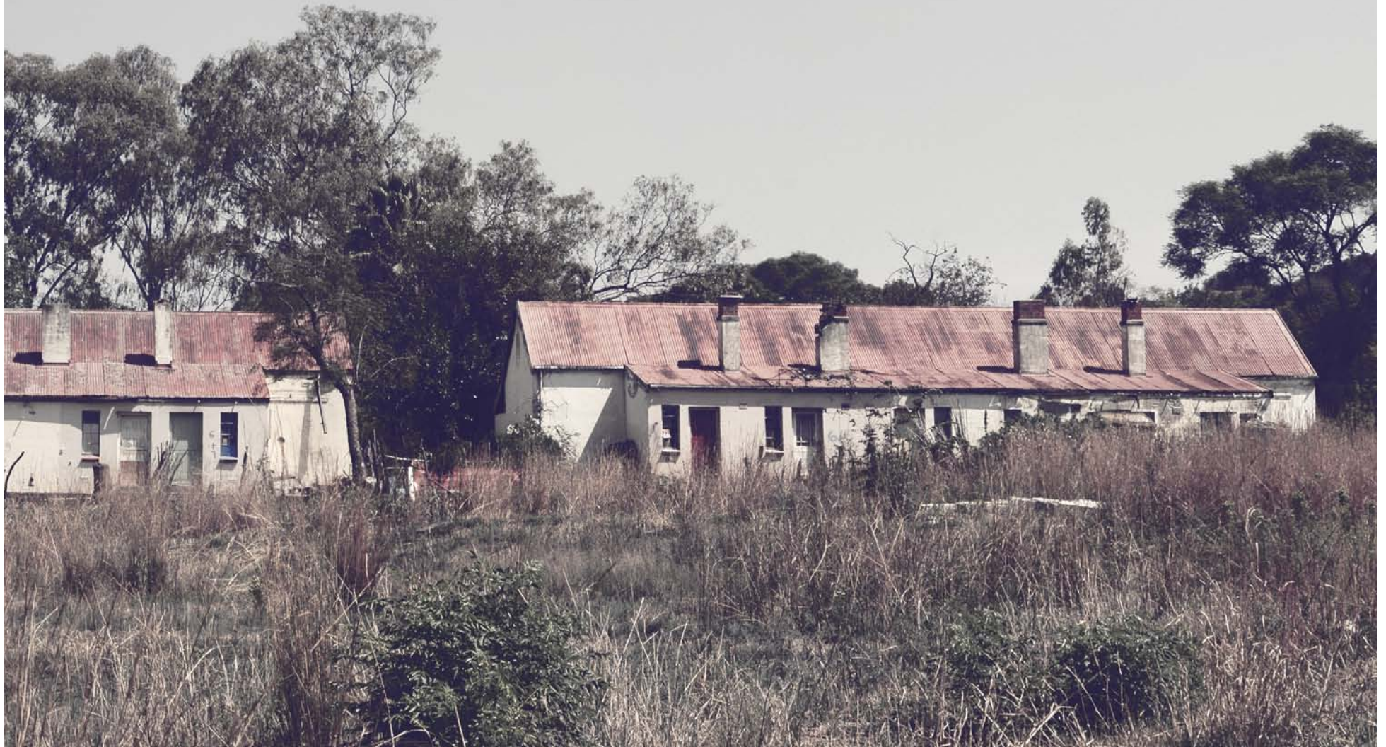
Illustration 1: Housing complex at Fort West in Pretoria West (Author, 2012).
