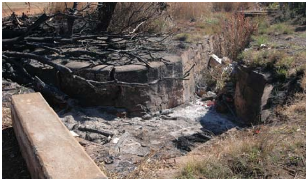
Illustration 41: Water furrows on site which forms part of the stormwater system (Author, 2012).
