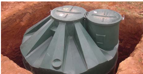
Illustration 157: Biogas converter.
