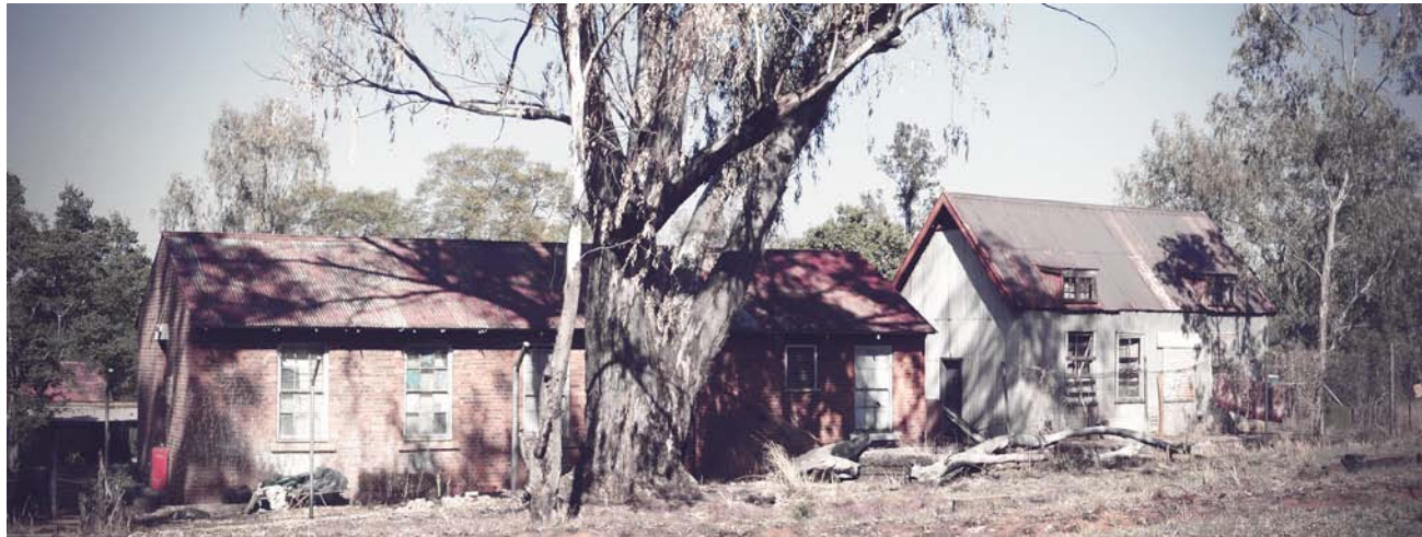
Illustration 35: Workshop buildings found at Fort West (Author, 2012).
