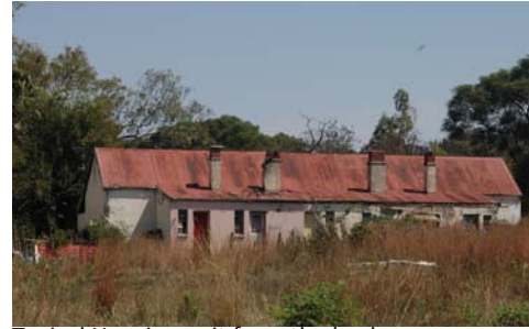
Typical Housing unit from the back
