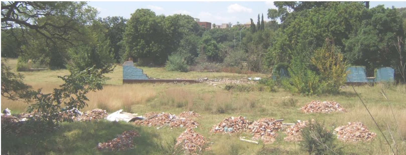
Fig. 61: Foundations of Demolished Buildings (Author, 2012)
