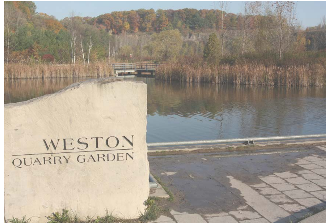
Fig. 83: Retention dam at Evergreen Brick Works (Young, 2011)
