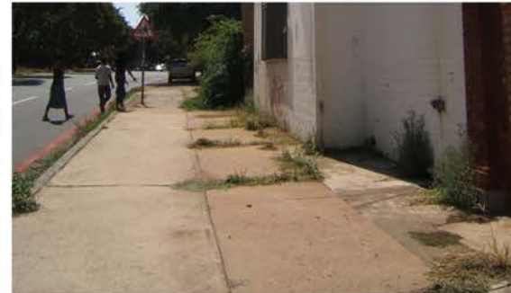
Reuse concrete slabs removed on site
