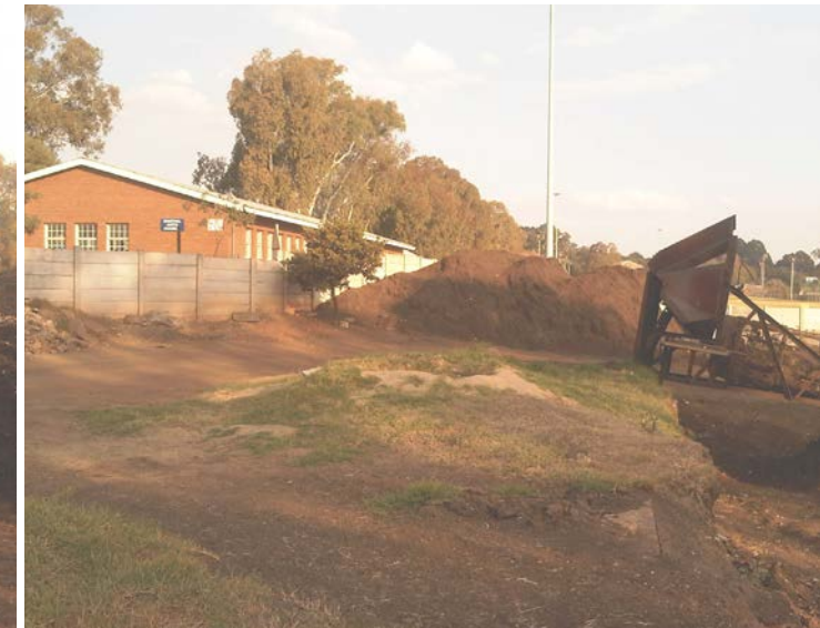
Fig. 97: WITS Composting Facility (Boshoff, 2012)
