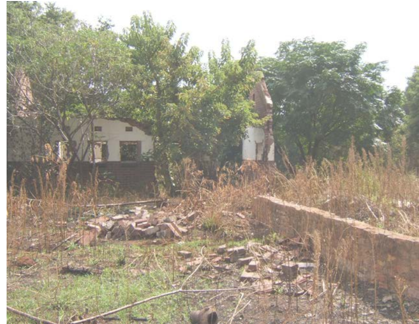
Fig. 63 & 64: Foundations of Demolished Buildings (Author, 2012)
