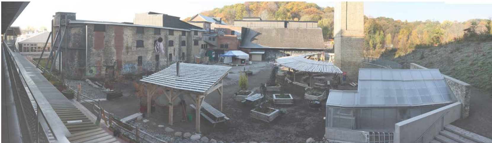
Fig. 78: Chimney Court (Young, 2011 modified by Author, 2012)
