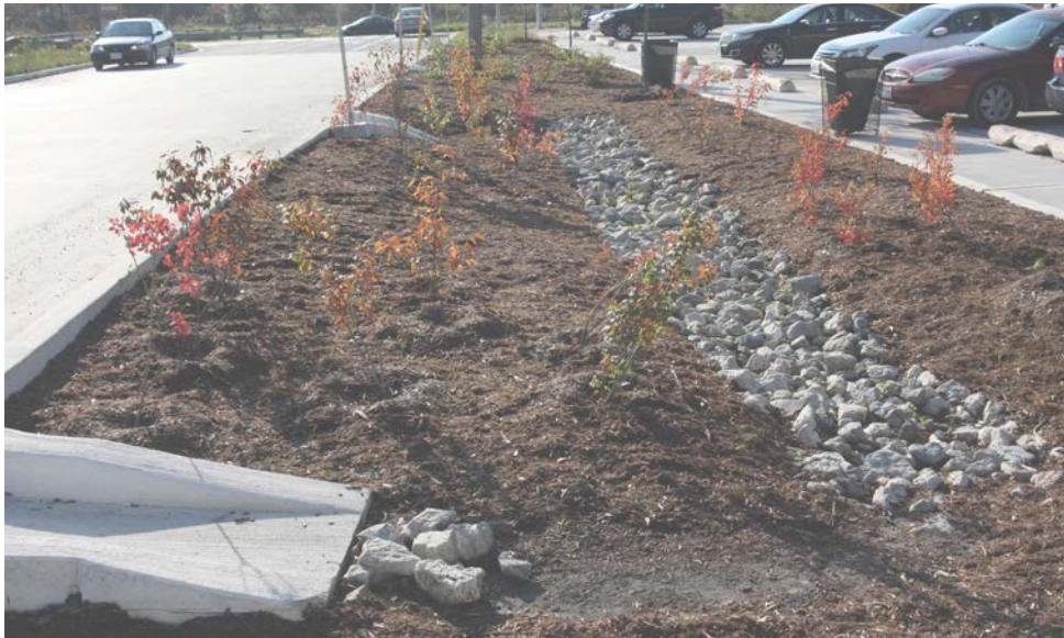
Fig. 79: WEST Parking lot at Evergreen Brick Works (Young, 2011)
