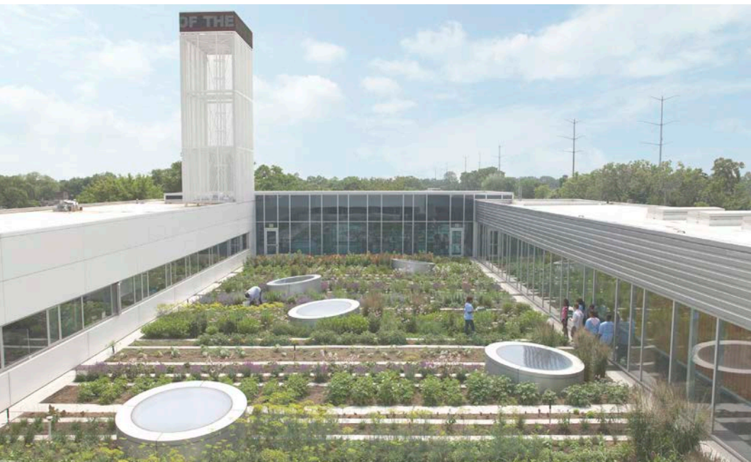
Fig. 103: Rooftop Haven for Urban agriculture (ASLA, 2010 photo by Shigley, S.)
