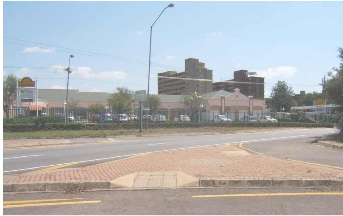
Fig. 54: Fountains Motown Shopping Centre (Author, 2012)
