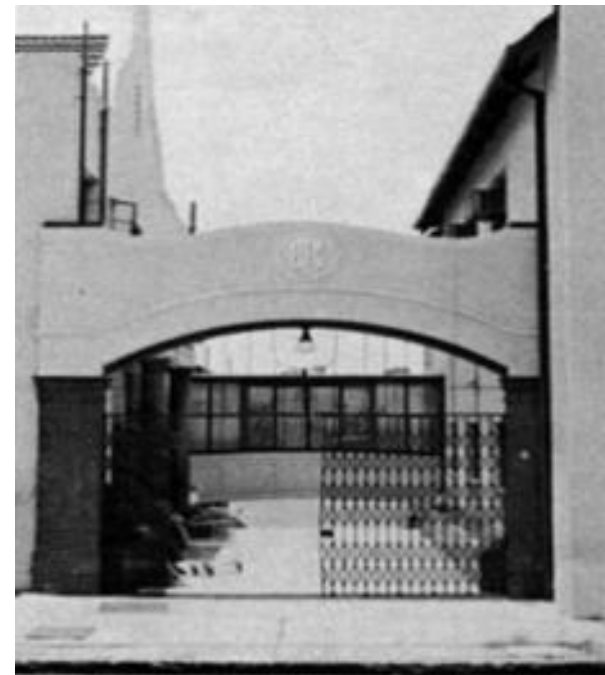
Fig. 49: Bridge connecting the Club House and Club Hall (Le Roux, 1992:156)
