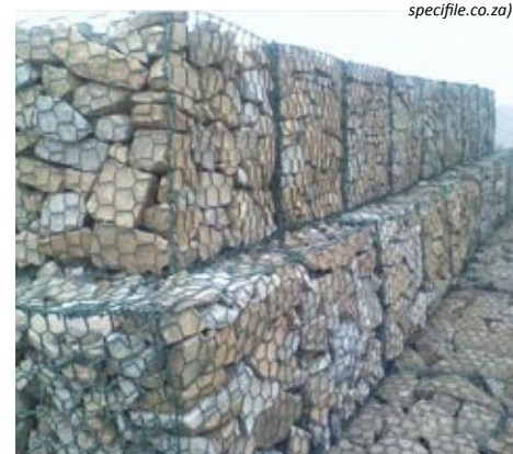
Illustration 241: Gabions filled with broken concrete (From: http://nitinwirenetting.com/gabion_mesh )
