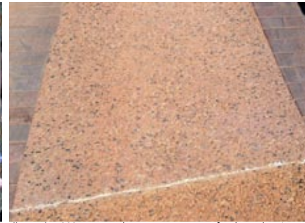
Illustration 233: Exposed aggregate concrete for the pedestrian and cycling pathways (Author, 2010)
