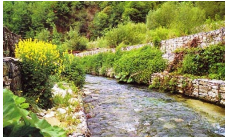
Illustration 37: Latium gabion structures retaining the Farta Creek, Italy. A sense of ecology has been restored to this stream through the bio-engineering intervention (Maccaferri Gabions, 2001:14)
