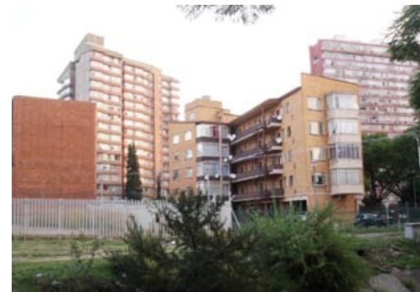
Illustration 61: Typical High rise flats of Sunnyside East (Author, April 2012).
