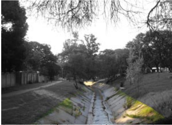
Illustration 99: The weed-infested concrete channel of the Walker Spruit at its base flow. Note the trapezoidal cross-section. (Author, May 2012)
