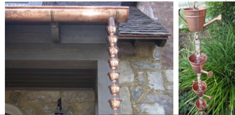
Illustration 203: Understanding the 'rain chain', a decorative alternative to a gutter downpipe which serves as inspiration for a falling water feature from the aqueduct to ground level (From: TheFunTimesGuide.com ).
