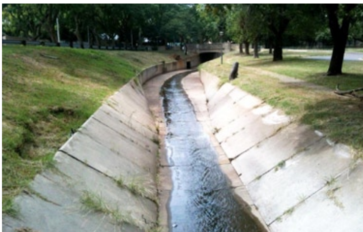
Illustration 36: The canalized Walker Spruit shows no sign of ecology (Author, April 2012)
