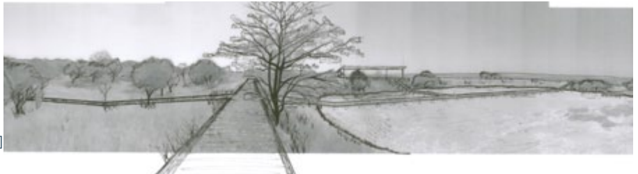
Fig. 6.12: [7] Restaurant and Dam. [Author, 2012]
