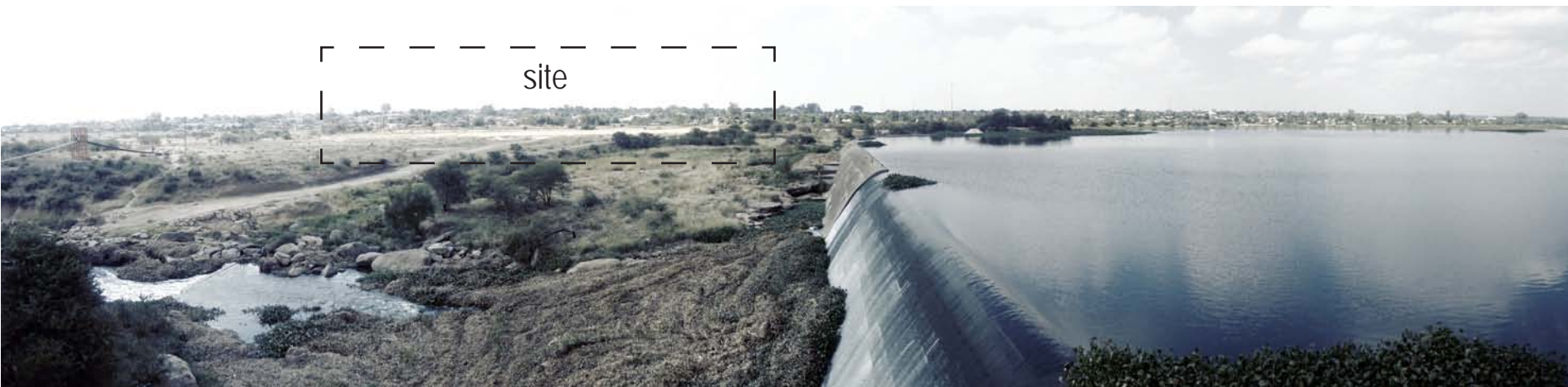
Fig 5|17_ View from Leeuwkraal Dam wall, Author 2012
