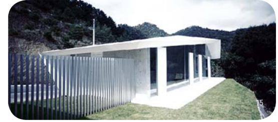
F House, 2011 Katsufumi Kubota Architect Yamaguchi, Japan
