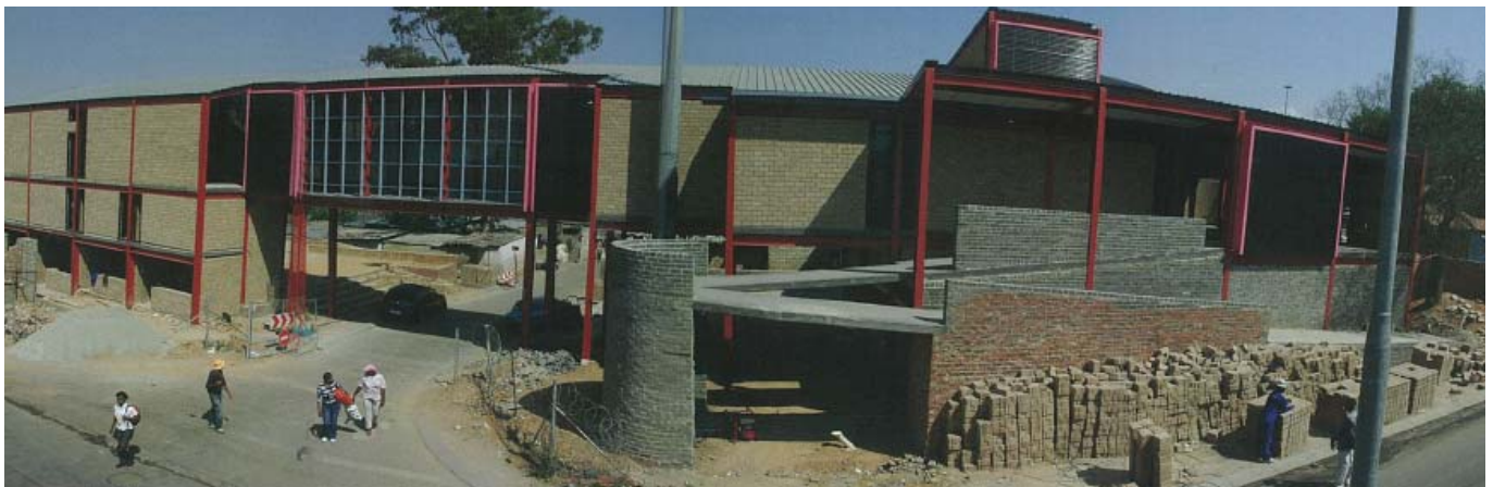
Figure 5.7: Photograph of facade during construction.
