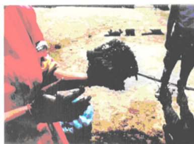
Figure 6.4 The method of mixing and preparing the earth and cow dung mixes
