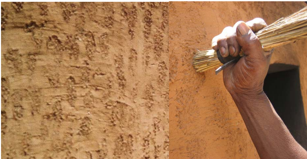
Figure 4.4 The tool used to indent the earth was a bundle of grass. Shade made it legible
