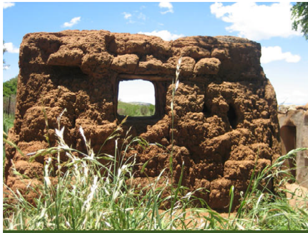
Figure 6.9 Earth blocks or sods were used as alternative to the use of a sapling frame
