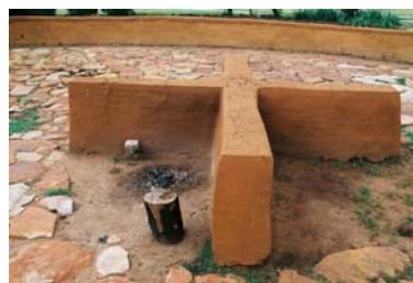
Figure 5.26 Cross shaped walls orientated to counter wind direction
