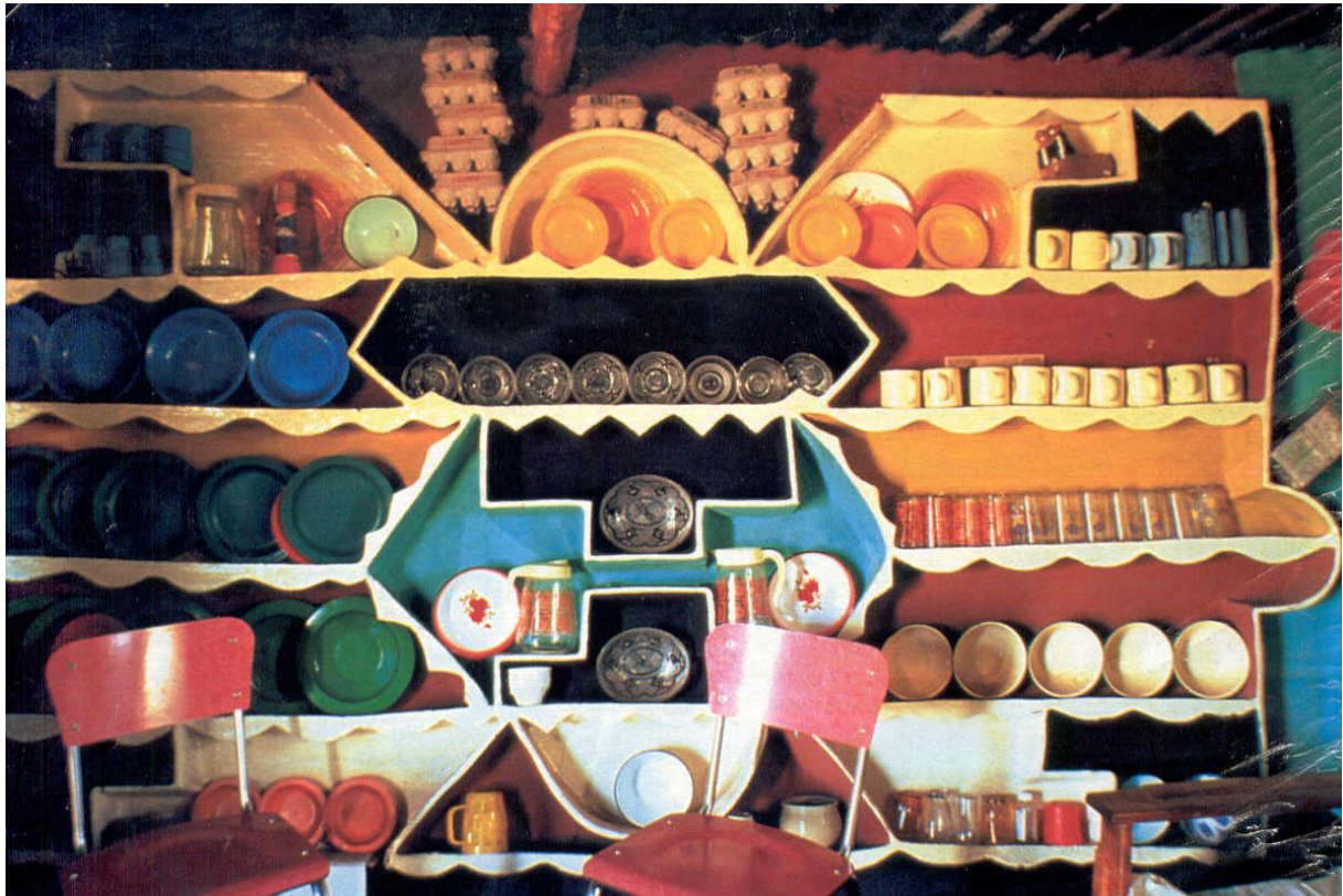
Figure 5.43 A vertical shelf made of earth
