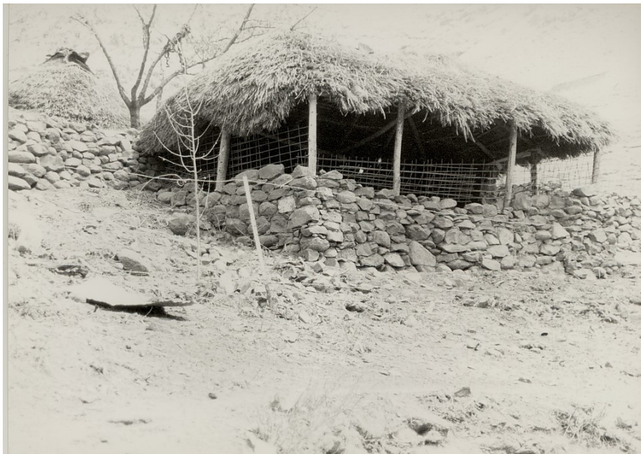
Figure 5.14 The animal kraal and kgotla ; walls were also of dry packed stone
