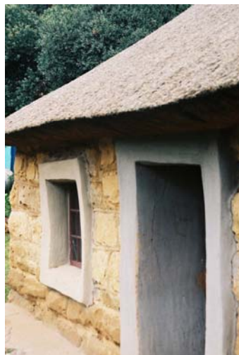
Figure 5.20 Surrounds to openings were a haptic necessity
