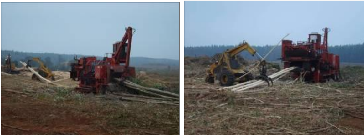
Figure 17: Trees being fed into the CFDD, and Figure 18: The Bell loader removing trees
