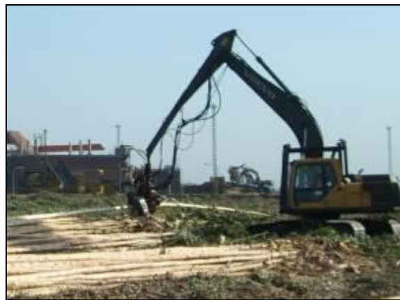
Figure 25: The DHP in operation
