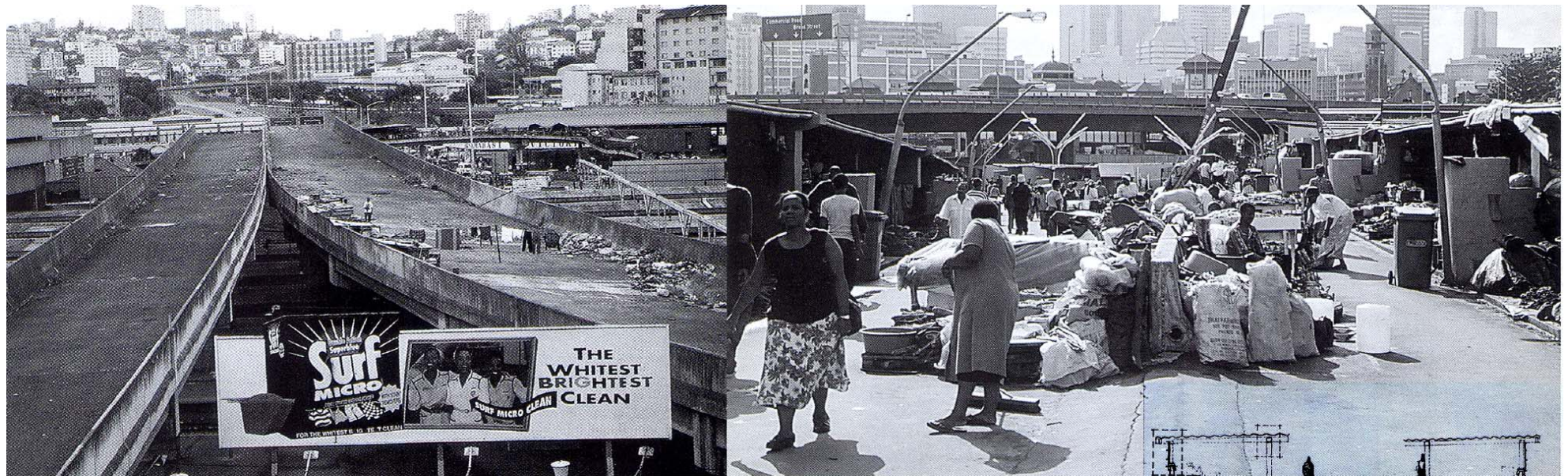
Fig 45: Market Road Bridge
