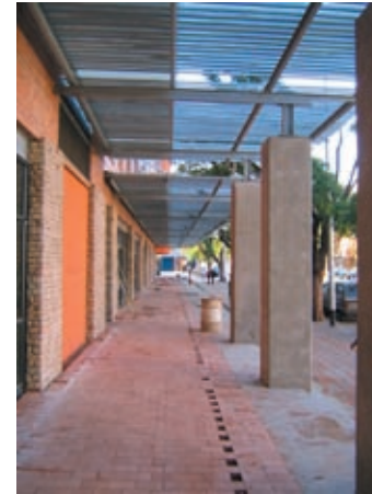
FIG. 5.2.4.4 Colonade at the new DTI Campus in Sunnyside
