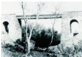
FIG. 5.3.2.7 NZASM Apies River bridge on the Eastern Line east of Salvokop
