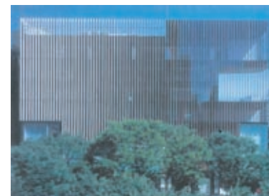
FIG. 5.3.4.1.2 example of vertical louvres on the exterior of a building
