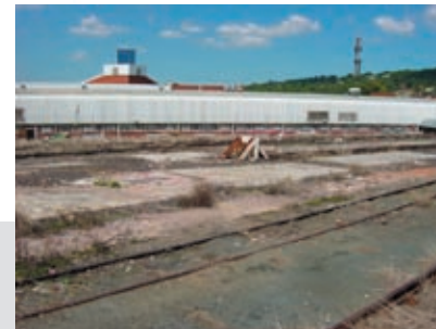
FIG. 5.2.5.4 Existing rail on site
