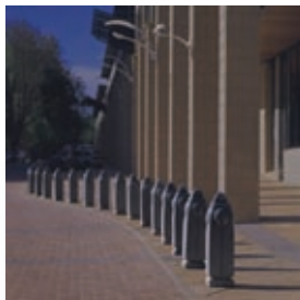
FIG. 5.2.2.2 Bollards at Melrose Arch
