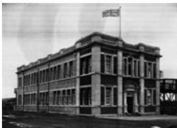
FIG. 5.3.2.2 CSAR Chief Mechanical Engineers Office of 1909. Massing of the structure provided thermal control by keeping the building cool in summer and relatively warm in winter
