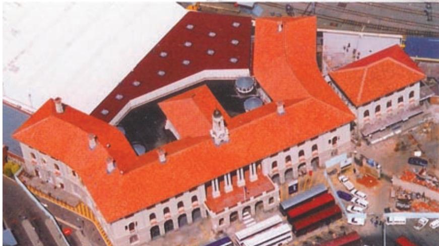
FIG. 1.5.34 Aerial view of Pretoria Station building showing the low pitched roof
