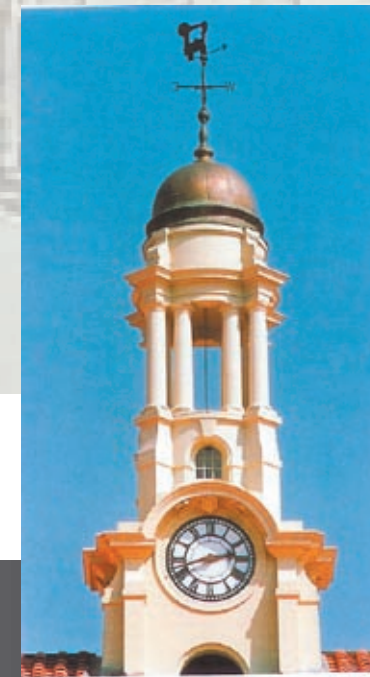
FIG. 1.5.49 Image of the clock tower after restoration
