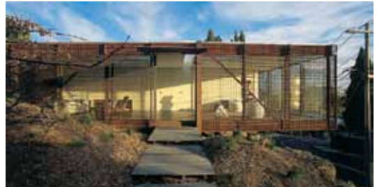
Figure 213 - image of similar stainless steel cladding used in Kew House, Melbourne, Australia by Sean Godsell 1996-1997.
