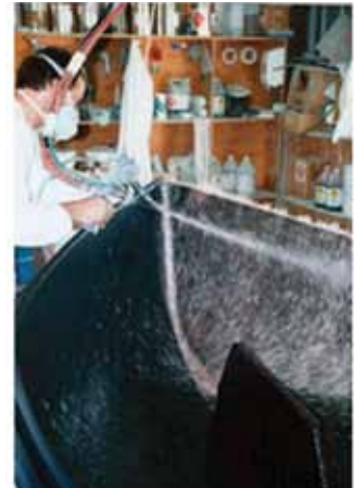
Figure 209 - image of first layer of fibreglass being sprayed on.
