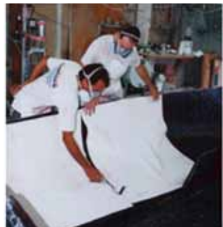
Figure 210 - image of 'core' material being added for stability and bulk.
