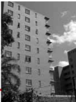
Figure 147 - image of residential blocks.
