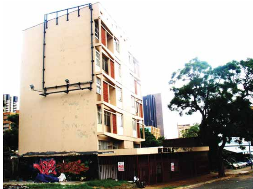
Figure 5.4 (below) The Berrals building - A 5 storey apartment block isolated on the urban island (Author, 2010)
