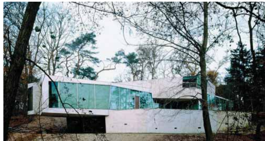
Figure 5.43. (bottom) Exterior view (UNStudio, 2010).
