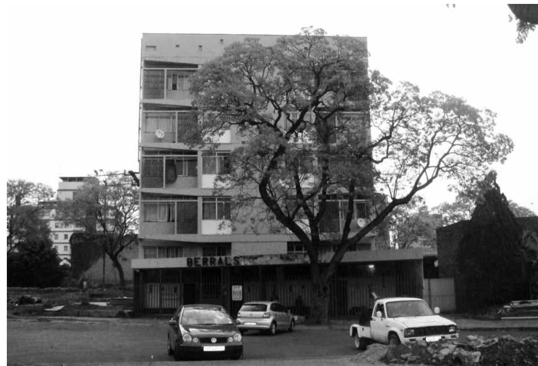
Figure 6.38. (below) The Berrals building - Eastern facade with the brise soleil screen (Author, 2010)
