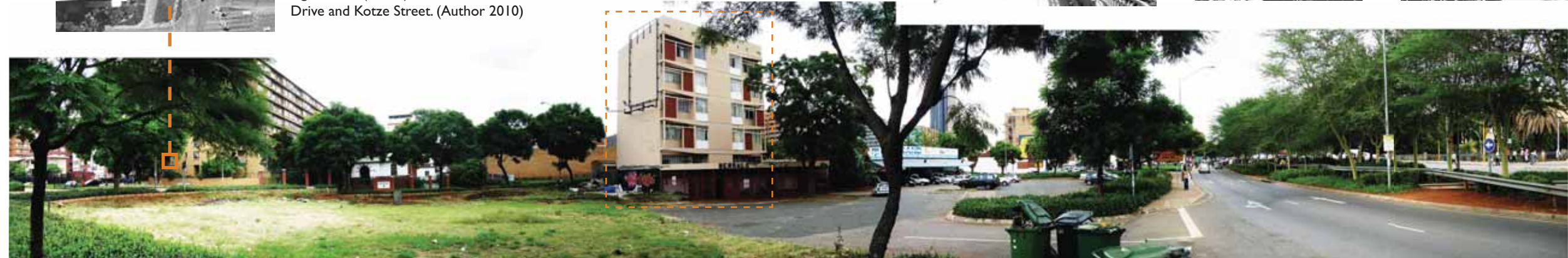
Figure 5.12. (below) - Corner of Nelson Mandela Drive and Kotze Street. (Author 2010)
