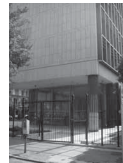
Figure 4.3. Palisade fencing used to block access to space that was once public (Author 2010)
