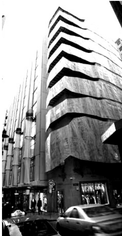
10. FUNCTIONING OF CH2 BUILDING (AUTHOR 2010).
