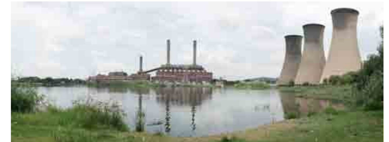
fig. 57_ Pretoria West Power Station with the dam in the foreground
