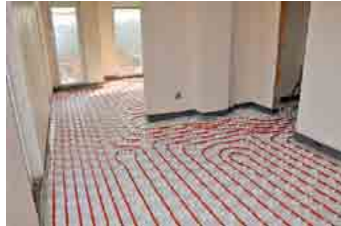
fig. 152_ Diagram illustrating the heating and cooling pipes
