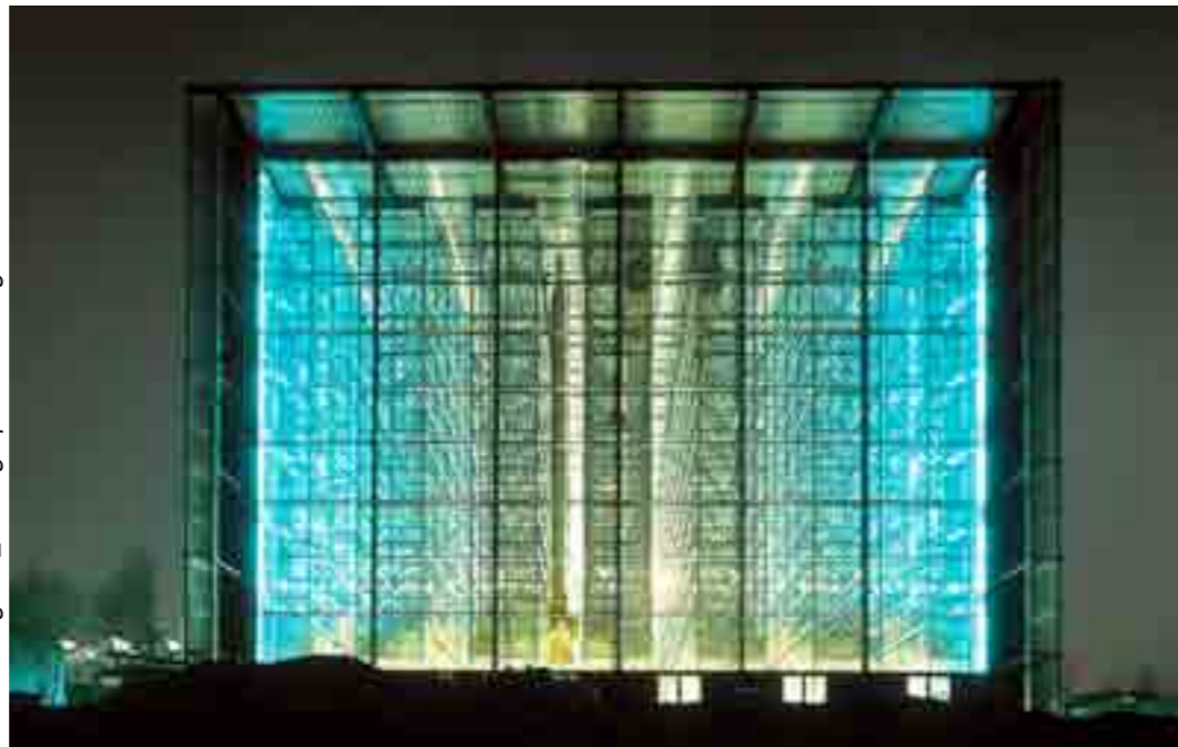
fig. 84_ Photograph of building exterior
