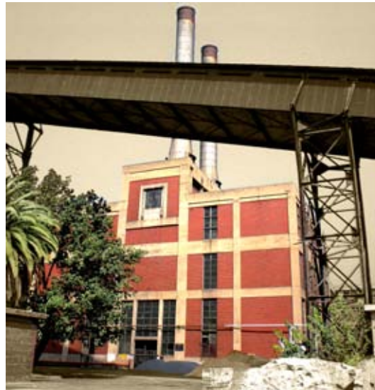
fig. 77_ East Elevation showing entrance and the buildings form
