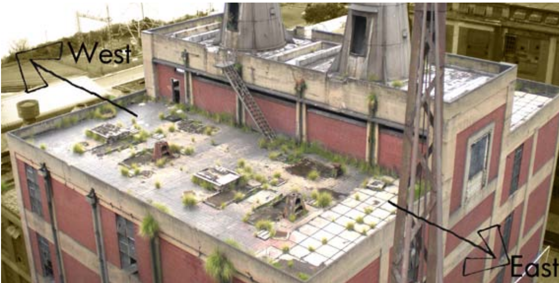
fig. 88_ The Boiler House's roof, lends itself to beautiful views to the East and the West, the flat roof has the potential of becoming a roof garden or event space for the new furniture production workshop.
