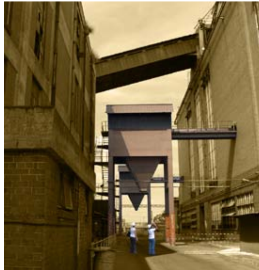
fig. 95_ A bridge will protrude through the ash hopper between Station A and Station B
