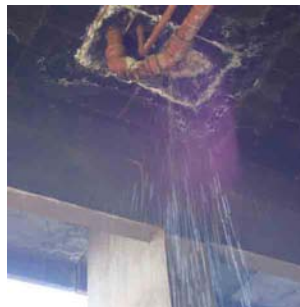
Fig. 5.21 Sewerage leaking from damaged pipes
