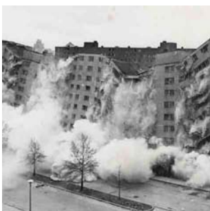
Fig. 5.25 Demolition of Pruitt-Igoe in 1972
