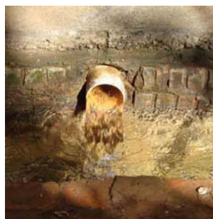
Fig. 5.22 Clear drinking water flowing from the building into the storm-water system
