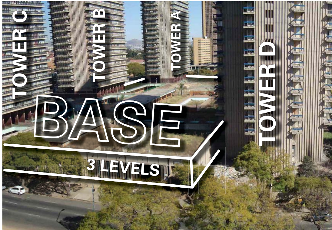
Fig. 5.39 Basic components of the Schubart Park complex
