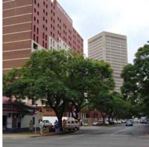
Fig. 4.6 Government and institutional office buildings
