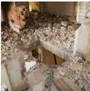
Fig. 5.16 Conditions within Schubart Park’s Tower D : Ducting and internal walls removed
