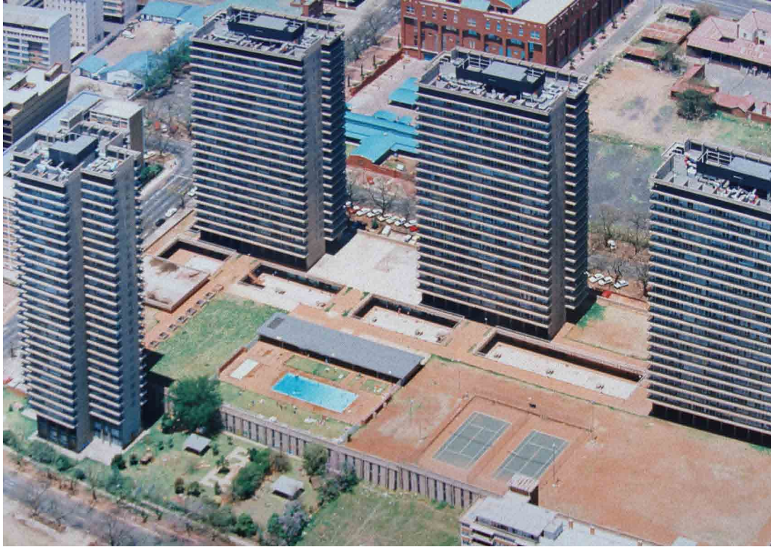
Fig. 5.3 Elevated view from the north-west
