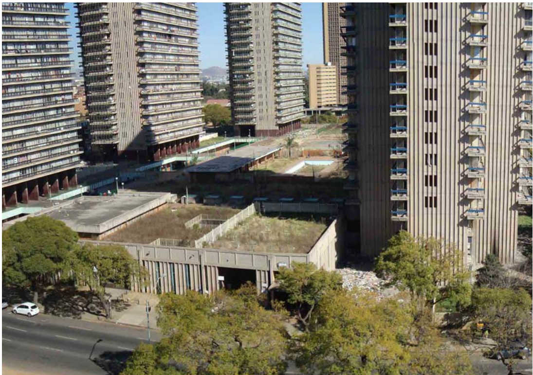
Fig. 5.2 View of Schubart Park from the east
