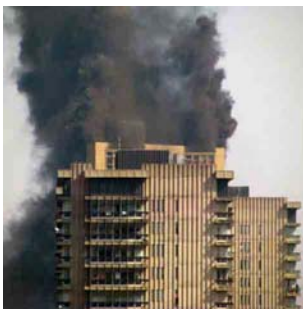
Fig. 5.12 On 22 July 2008 a fire was started in the Kruger Park building during attempted evictions at Schubart Park
