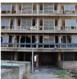
Fig. 5.18 Damage to Schubart park;s Tower D caused by vandalism and looting
