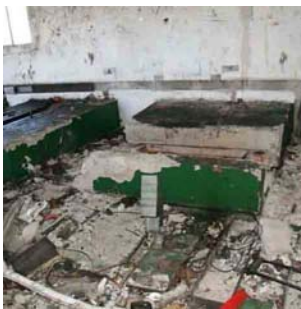
Fig. 5.15 Conditions within Schubart Park’s Tower D: Total destruction of lift-room
