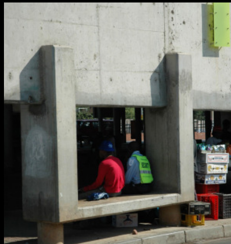
Figure 60. Portion of concrete spine acting as edge and seating
