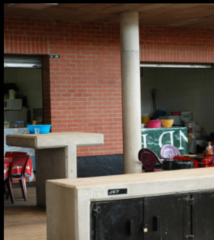
Figure 63. Internal view with pre-cast concrete furniture
