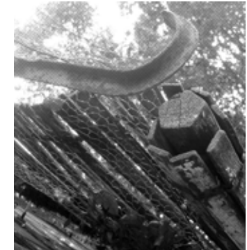
Fig_107: Roof detail with timber louvers.
