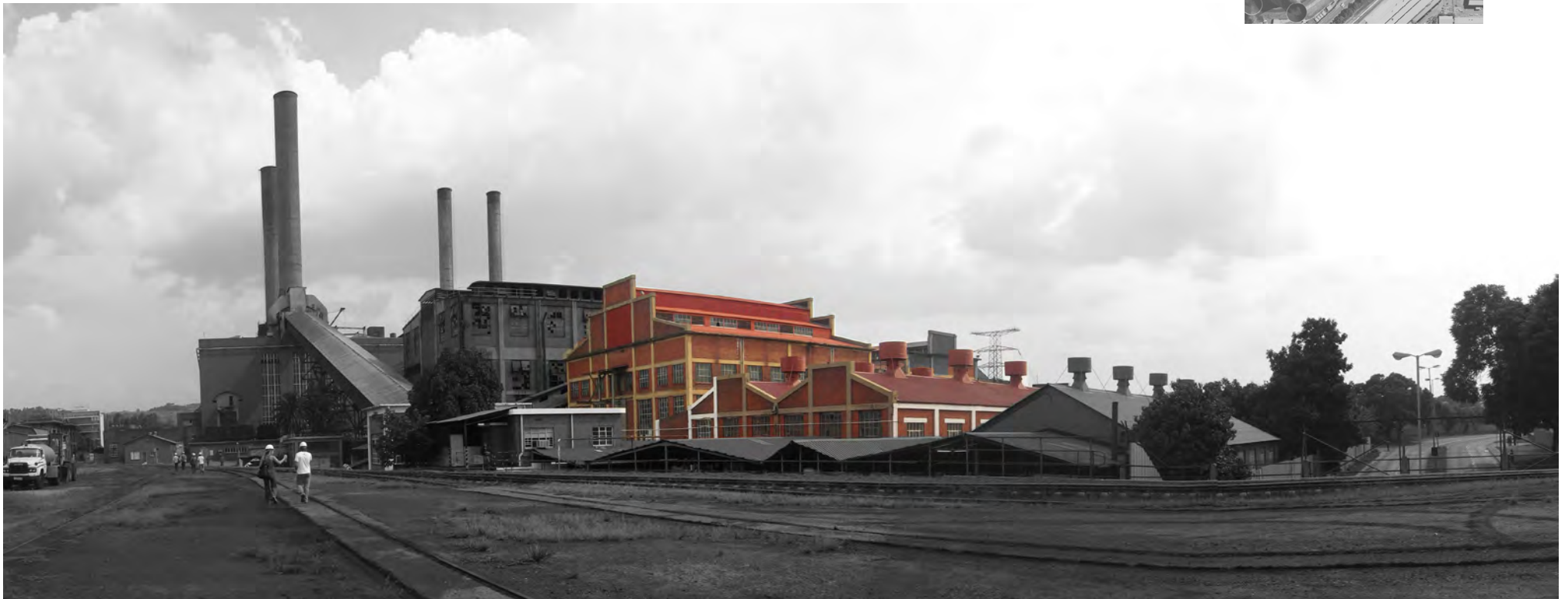
Fig 4.12 View of existing 1924 Boiler House and Workshop buildings in surrounding context
