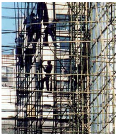
1. bamboo scaffolding & construction
