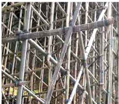
1. bamboo scaffolding & construction
