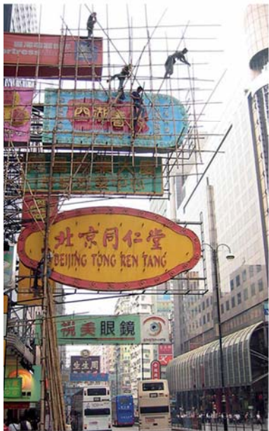
1. bamboo scaffolding & construction
