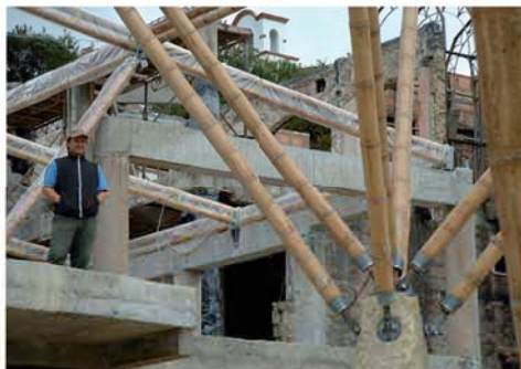
5. bamboo as structure column
