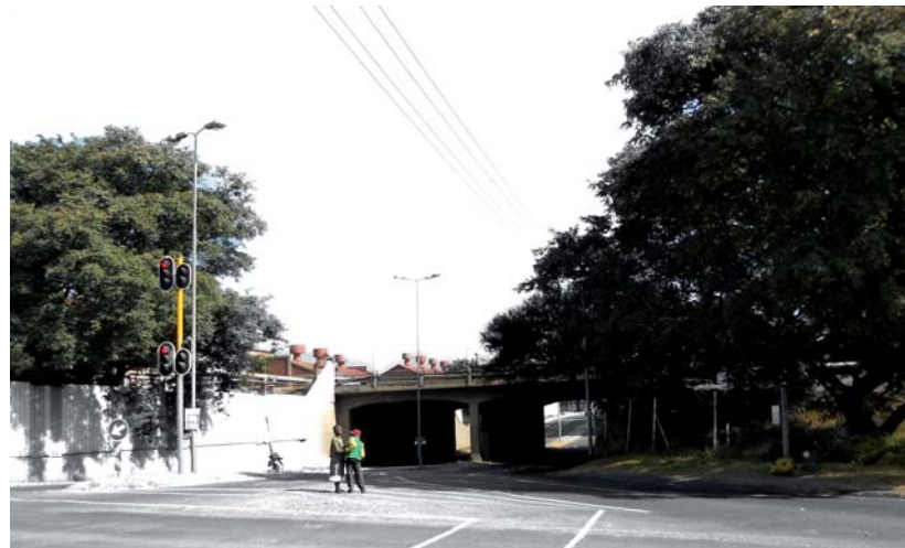
the railway bridge
