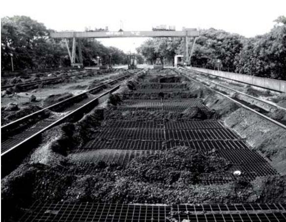
Figure 45 : On top of the bunker
