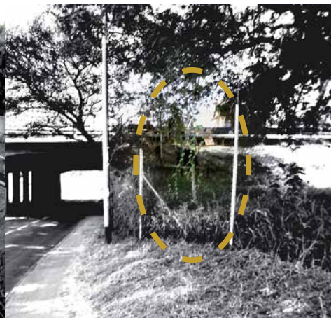
Figure 46,47 : Steel steps down to Buitekant Street
