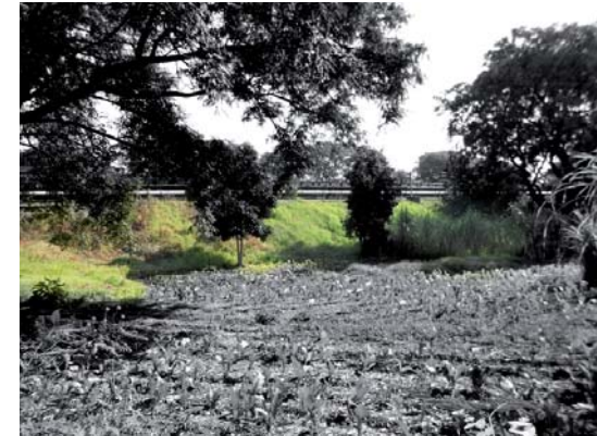
Figure 50: The old coal bunker is buried by vegetation [author, 2010].
