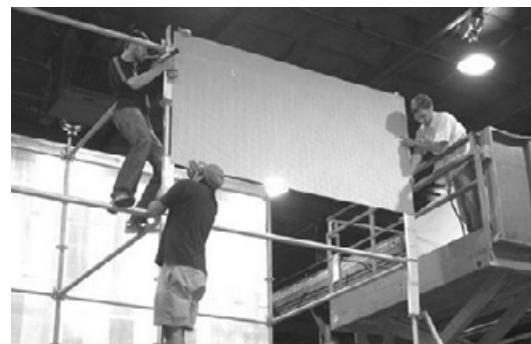
Figure 119. Eight volunteers assembling the media wall (Arquitectura de Interiores, 2008).
